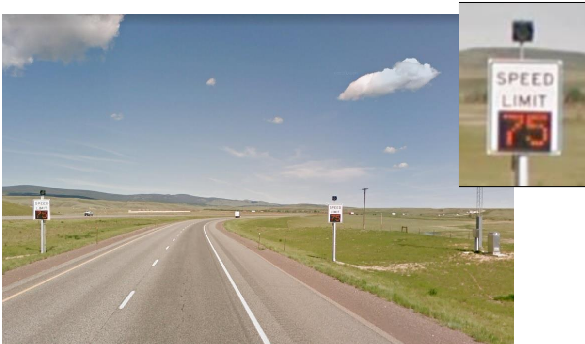
Figure 17. WYDOT IH 80 Variable Speed Limit Installation.
