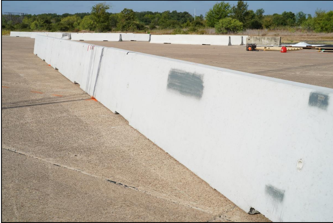
Figure 3.6. Downstream View of the Flared Single-Slope Portable Concrete Barriers prior to Testing.
