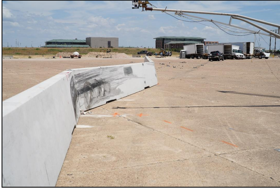
Figure 6.5. Flared Single-Slope Portable Concrete Barriers after Test 440862-03-3.
