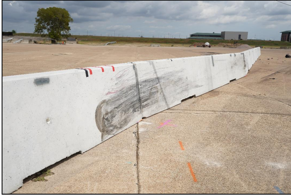
Figure 7.5. Flared Single-Slope Portable Concrete Barriers after Test at Impact Location, Test 440862-03-4.
