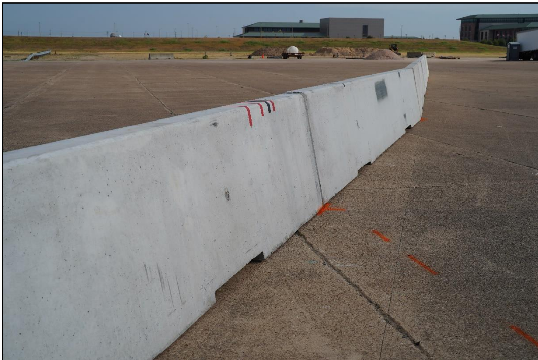
Figure 3.3. Flared Single-Slope Portable Concrete Barriers at Impact Prior to Testing.
