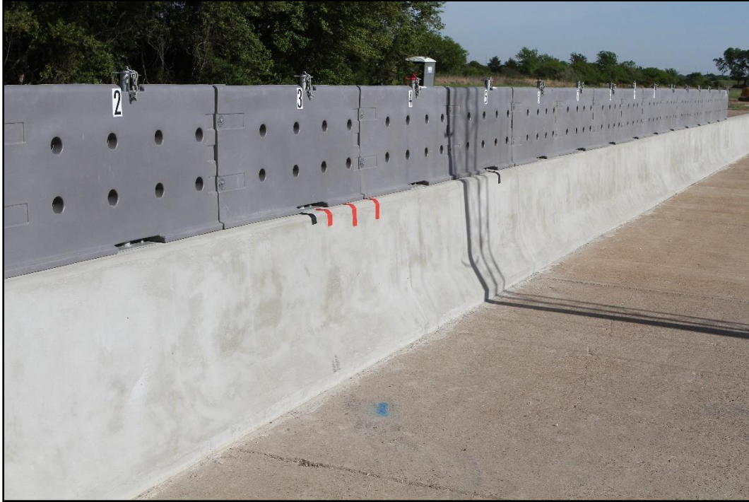
Figure 2.10. The Armorcast® Gawk Screen on F-Shape Barrier prior to Testing.
