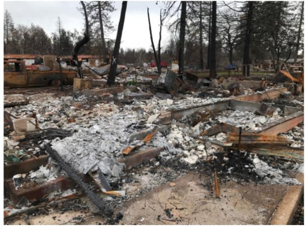
(b) Structures burnt by fire
