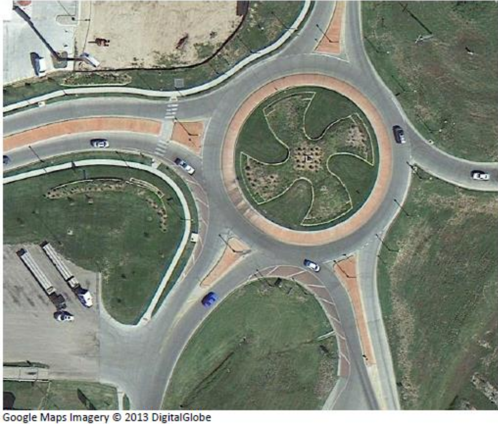
Figure 14. Striped Outside Truck Apron at the Intersection of I-70/S East Street/E Chestnut Street/E Ash Street in Junction City, Kansas (reproduced from Exhibit 6-48 in 15).
