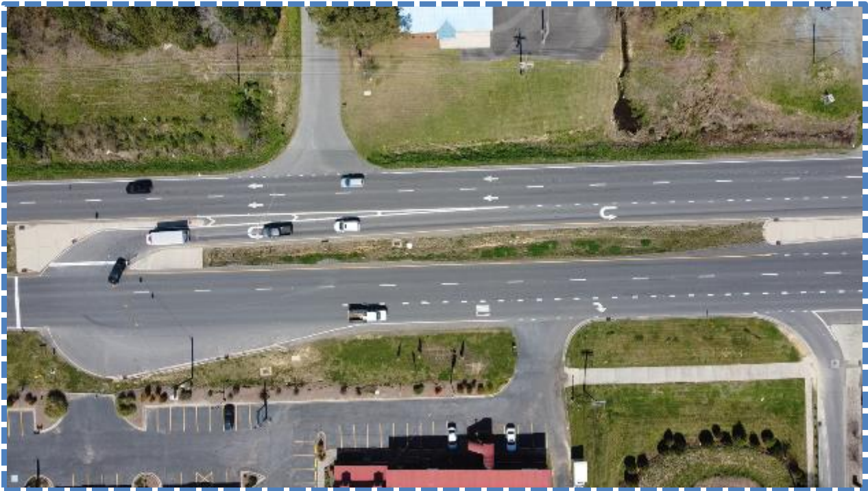
Figure 59. West U-Turn Intersection Camera View at Sardis Church Road Site.
