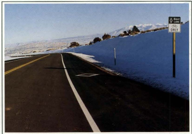
Signs alert motorists of nearby bicycle traffic.
