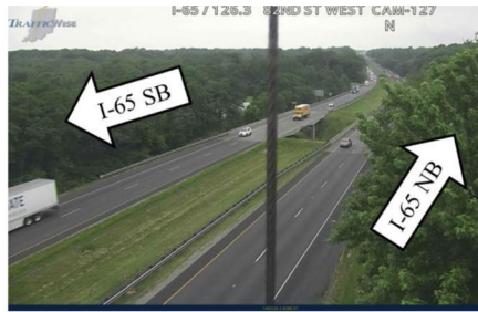
(a) Before very heavy rain at 10:36 AM at MM 126.3
