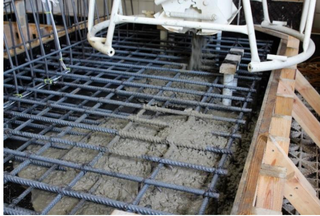
Figure 7-4 Deck concrete placement
