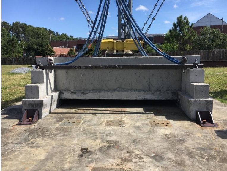
Figure 7-10 Backside of impact specimen after being positioned onto the pendulum foundation (with temporary HSS lifting element still connected)
