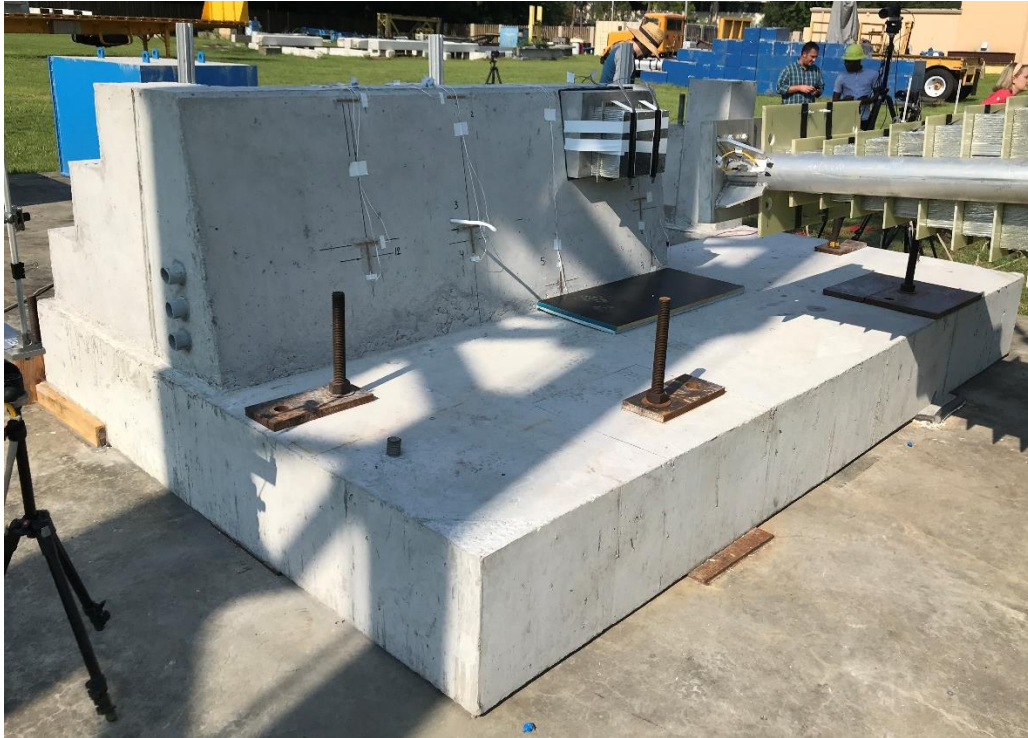
Figure 9-21 GFRP EOR specimen prepared and ready for pendulum impact testing (with instrumentation in place)
