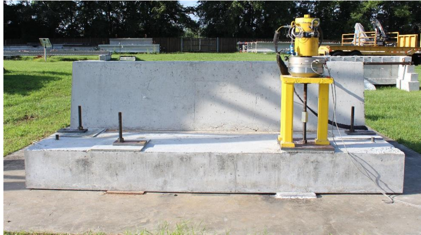
Figure 7-12 Post-tensioning fourth (front right) threaded bar for anchoring test specimen to pendulum foundation with the FDOT loading assembly
