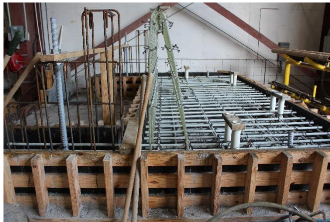
Figure 7-3 GFRP bars positioned inside deck formwork for GFRP bar reinforced specimen
