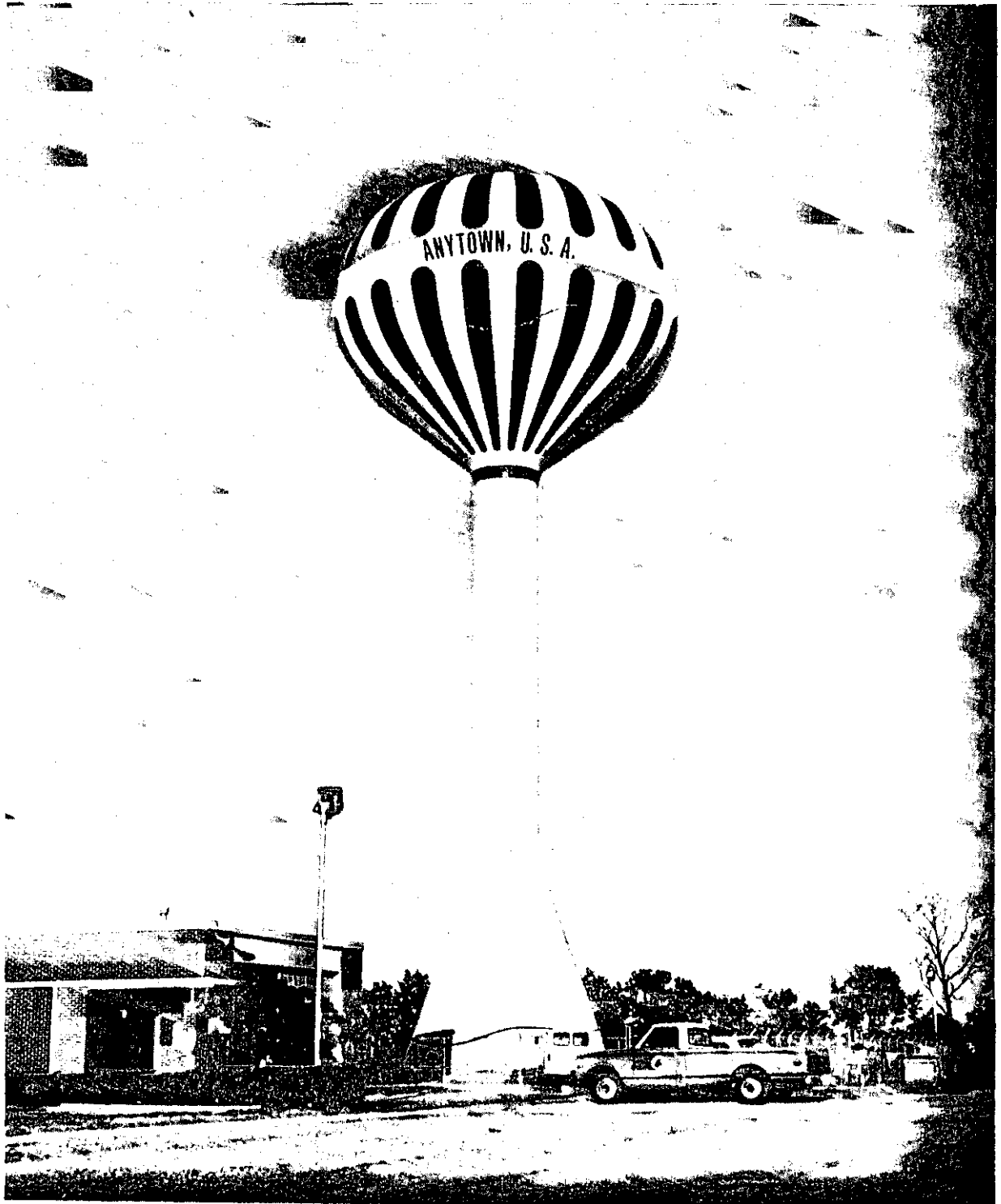
PAINTING OF SINGLE PEDESTAL WATER TOWER BY BEACHBALL PATTERN
