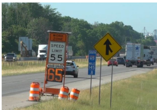
Figure 4.1 Radar-based speed limit sign with motorist speed feedback placed at I-65 southbound near MM 145.8.
