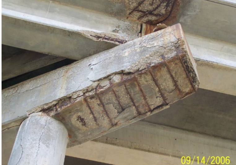
Figure 1.3: Leaking issues associated with expansion joints (Hyzak, 2021).
