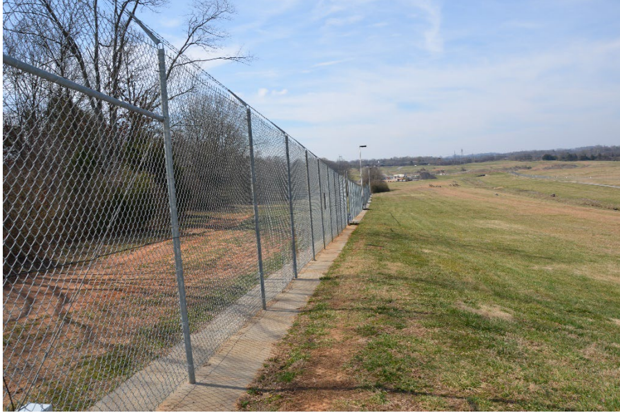
Figure 44. Fence Line in the Safe Skies PTF
