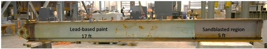
Figure 3.2 Girders sandblasted up to 5 ft. from the girder end.
