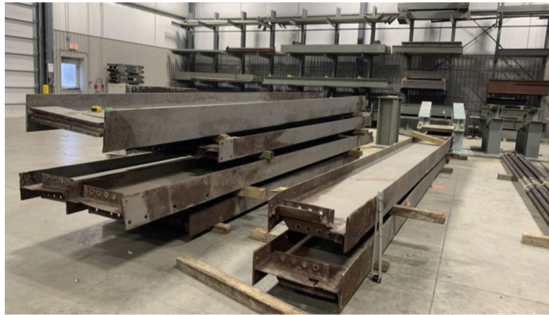
Figure 2.6 Corroded girders being stored at Thomas A. Page Pavilion at Purdue University.
