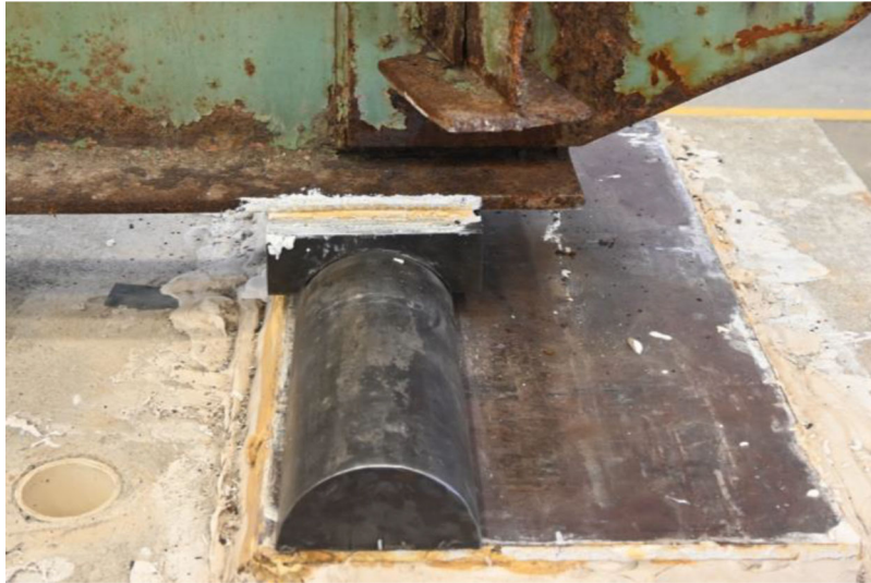
Figure 4.19 Simple support at the girder end.
