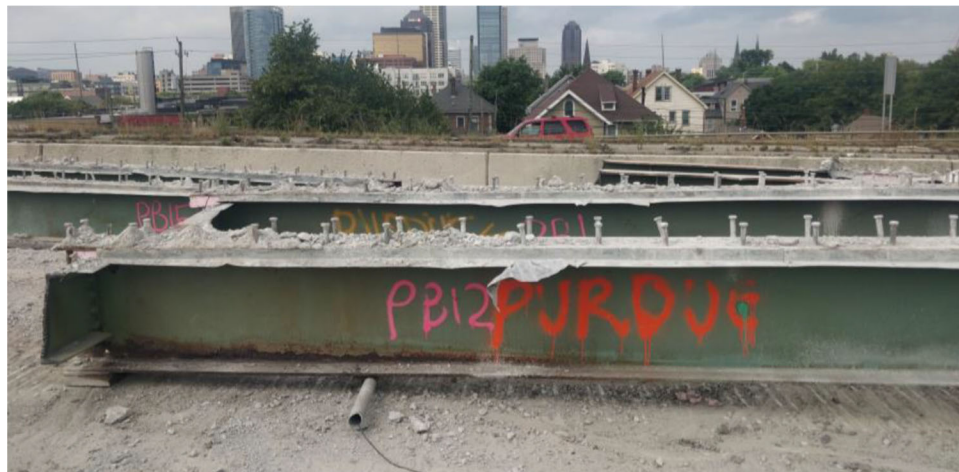
Figure 2.4 Girders temporarily stored on-site (courtesy of HNTB).
