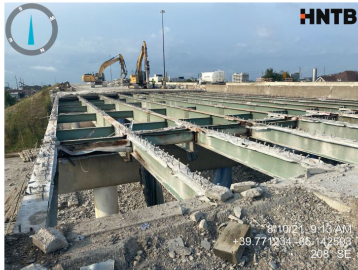
Figure 2.3 Concrete deck demolition (courtesy of HNTB).
