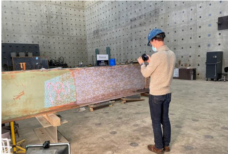
Figure 3.22 3D scanning of corroded girder.
