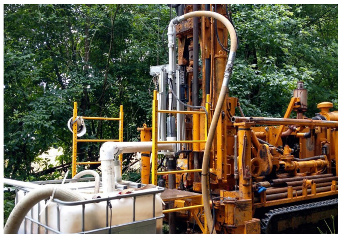
■ The ISTD equipment assembled in front of the drill rig.
