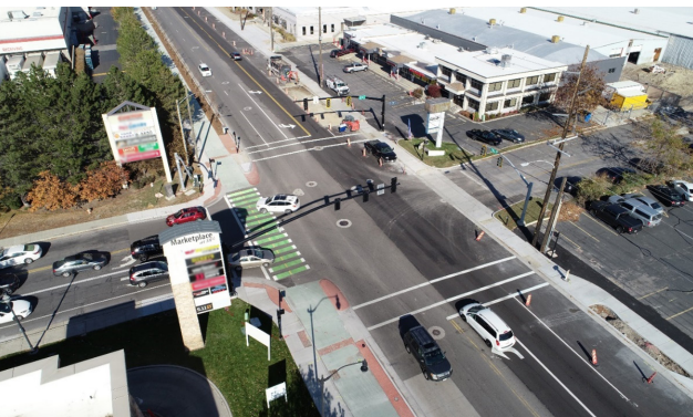
Figure 3. Photo. A roadway segment on 300 West Street after improvement.
