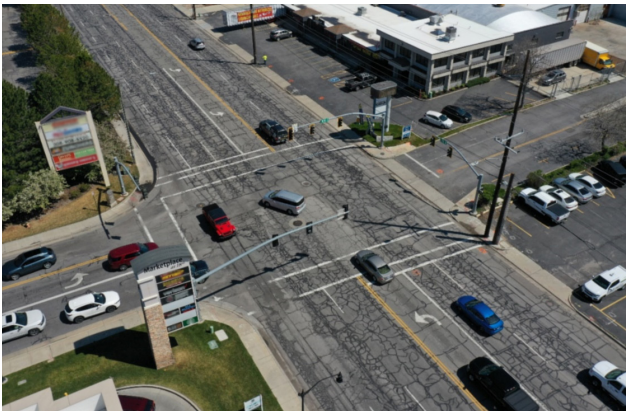
Figure 2. Photo. A roadway segment on 300 West Street before improvement.
