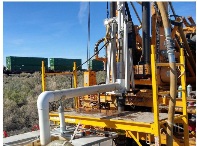
■ The ISTD equipment assembled in front of the drill rig.
