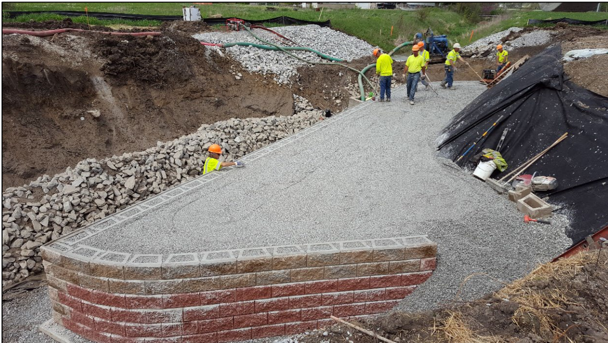
Figure 1. Photo. OGAs as structural backfill in a geosynthetic reinforced soil abutment.
