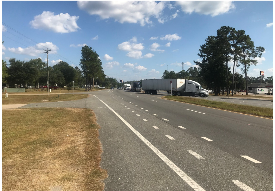
Figure 8. US-90 Midway project after treatment (Source: Gary Fitts).
