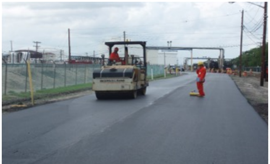
Figure 1. First-generation HPTO placement. Source: Dr. Tom Bennert
