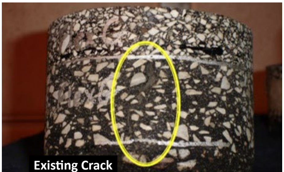
Figure 2. Core showing resistance to reflective cracking. Source: Dr. Tom Bennert
