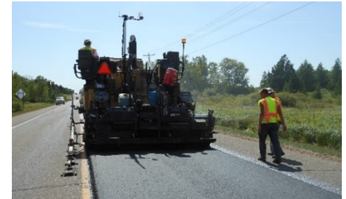
PMTP scans a highway paving job in Minnesota. Photo: MnDOT
