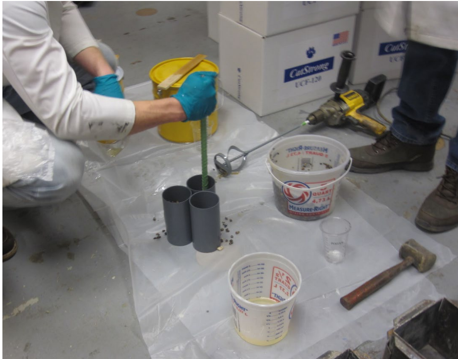
Figure 2.12 Preparation of Sikadur 52 Epoxy Mortar Compressive Strength Gain Specimens
