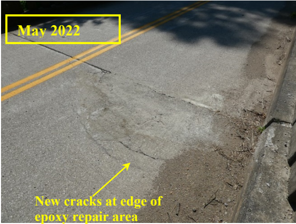
(a) Southbound lane over joint at Pier 1
