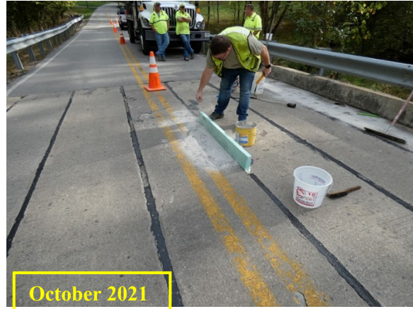
(b) Spreading Class I sand over repair area
