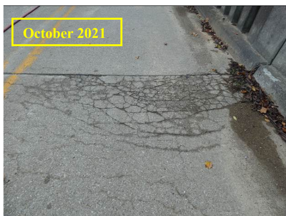
(a) Southbound lane over joint at Pier 1
