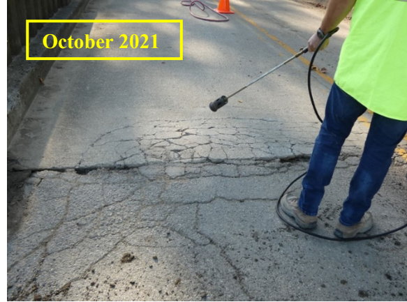
(b) Drying using blowtorch
