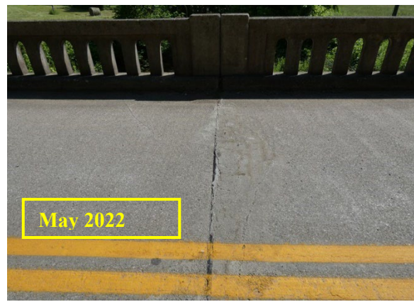
(d) Northbound lane over joint at Pier 2
