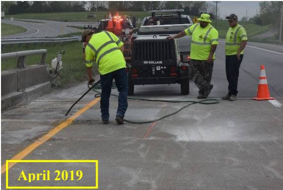
(a) Cleaning of repair area using compressed air
