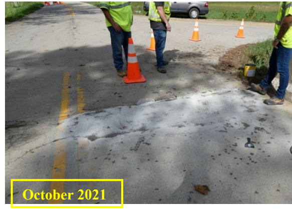
(b) Class I sand spread over epoxy
