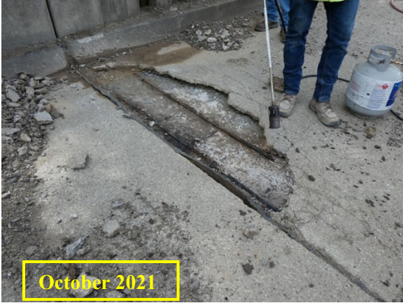
(a) Drying area after removing loose concrete
