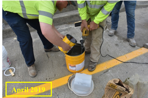
(b) Mixing of the two-part epoxy
