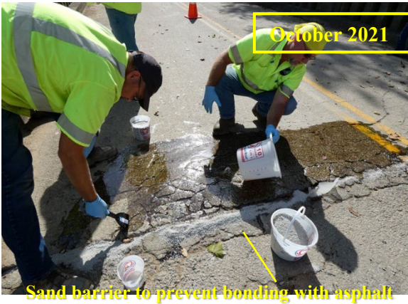
(a) Spreading of epoxy over cracked area
