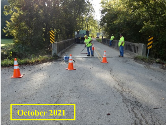
(a) Cleaning using compressed air
