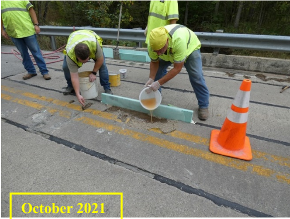
(a) Application of epoxy over pea gravel
