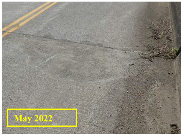
(c) Southbound lane over joint at Pier 2
