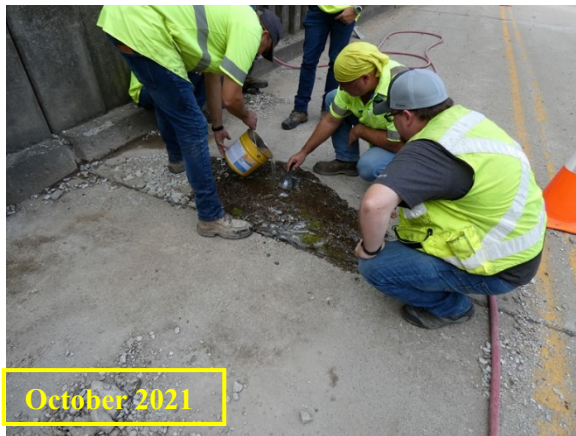
(c) Application of epoxy
