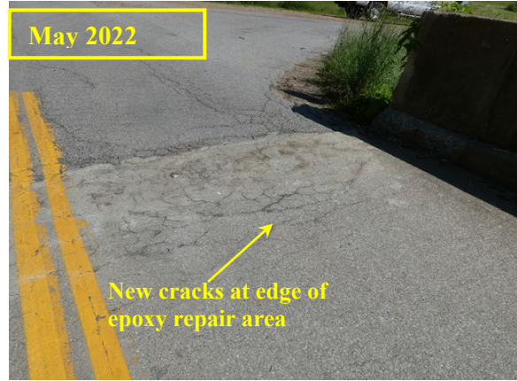
(b) Northbound lane at Abutment 2
