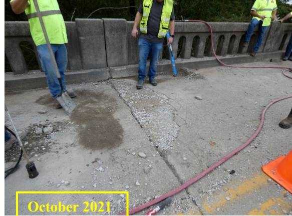
(b) Packing back removed concrete
