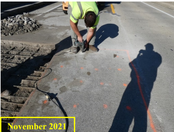
(a) Drilling of holes
