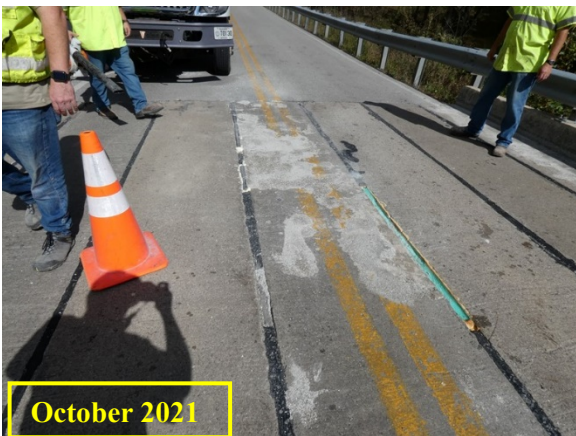
(a) Center PC beam soon after repair
