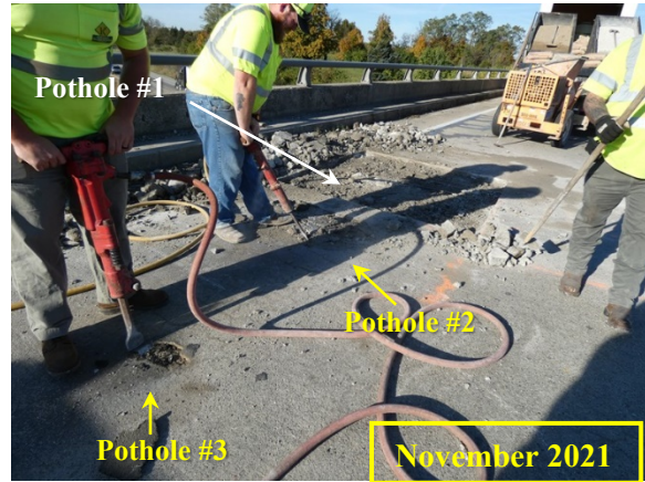
(b) Removal of damaged concrete in Pothole #2 and #3
