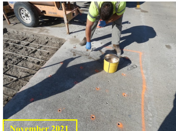
(b) Gravity feeding of epoxy
