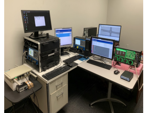
This connected vehicle-to-infrastructure applications environment setup tested wireless and wired connections for several CV applications.
