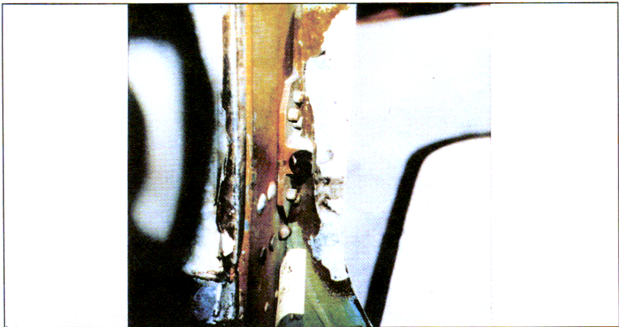
FIGURE 5-12. CORROSION DEVELOPED UNDER LEVELING COMPOUND INSTALLED DURING PREVIOUS REPAIR OF OVERWING EXIT
