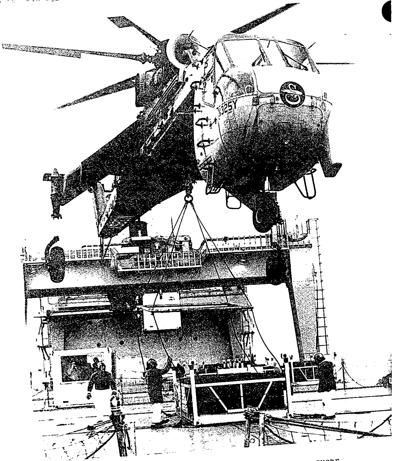
FIGURE 1-7. HELICOPTER MOVING CARGO FROM SHIP TO SHORE
