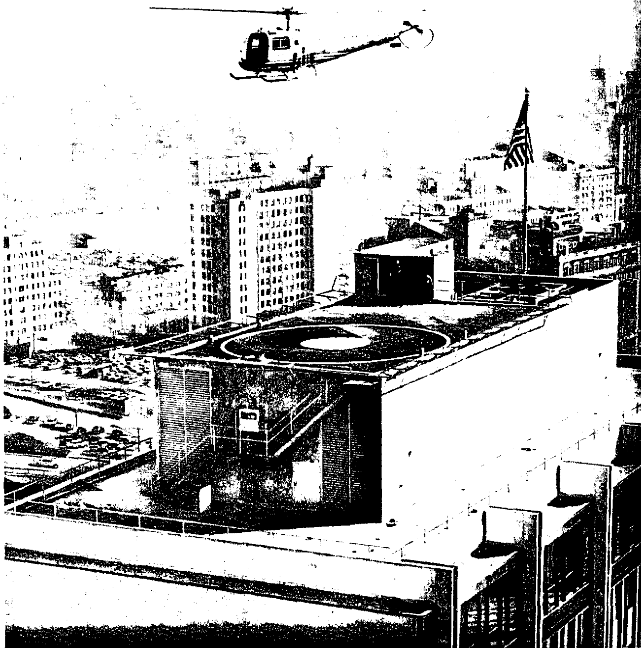
FIGURE 13. ROOFTOP HELIPORT, SIGNAL OIL AND GAS COMPANY, LOS ANGELES, CALIFORNIA, SHOWING CIRCLE MARKING AND HORIZONTAL SAFETY DEVICE EXTENDING FROM EDGES OF ROOFTOP
