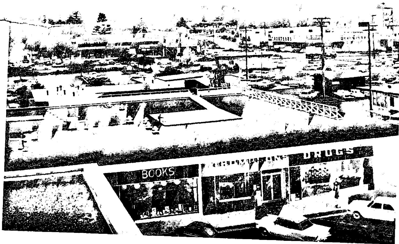
FIGURE 15. ROOFTOP HELIPORT, BELLEVUE, WASHINGTON, SHOWING 24' x 24' LOAD DISTRIBUTION PAD ON BUILT-UP ROOF AND HANDRAILS OR SAFETY BARRIERS
