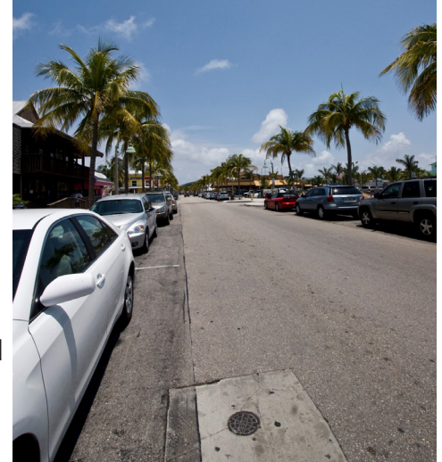
Superpave mixtures set for low traffic levels in Florida were recently tested for performance under heavy traffic levels.
