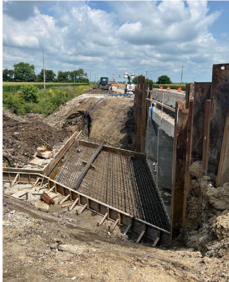
c) Box culvert demo project near Armstrong, Illinois
