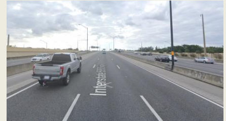
Managed lanes with concrete barrier separation
