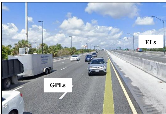
(a) Concrete Barrier Separation on I-595
