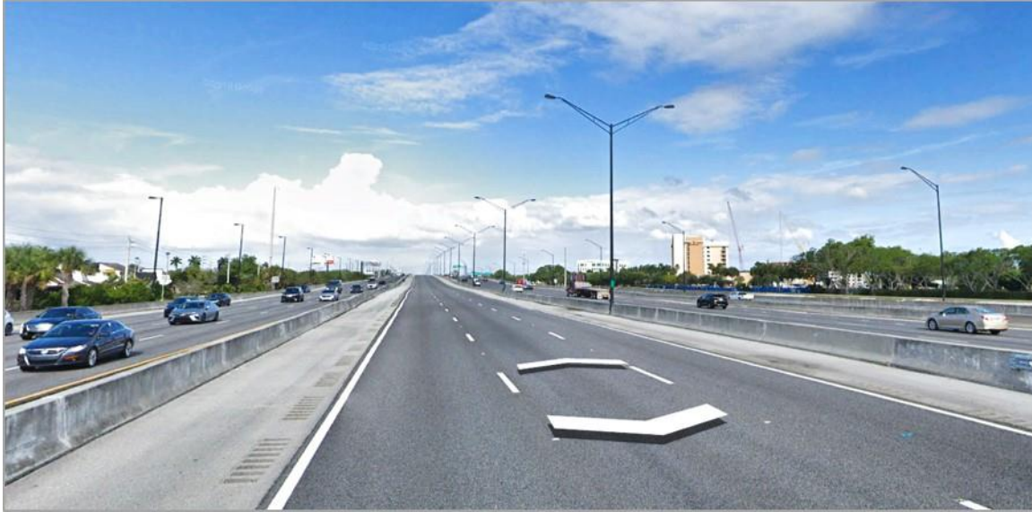
Figure 2.6: I-595's Reversible Lanes in Florida Separated by Concrete Barriers (Source: Google Earth)
