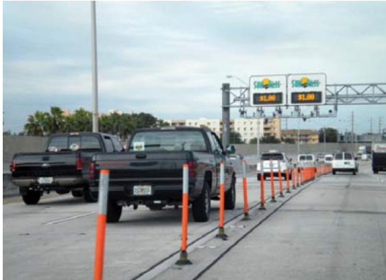
(a) Mountable Raised Curb Pylon Separation on the I-95 Express
