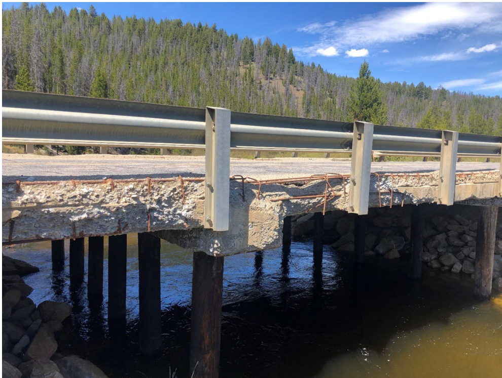
Figure 21: One of the Trail Creek bridges prior to replacement
