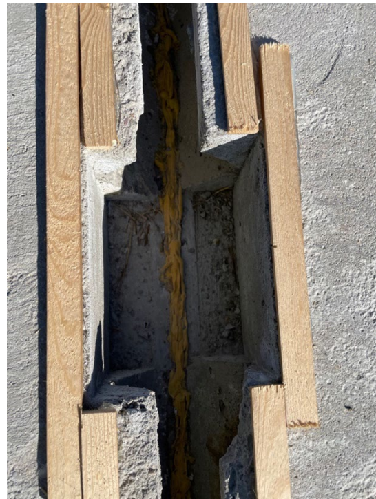
b) inside keyway showing foam sealant
