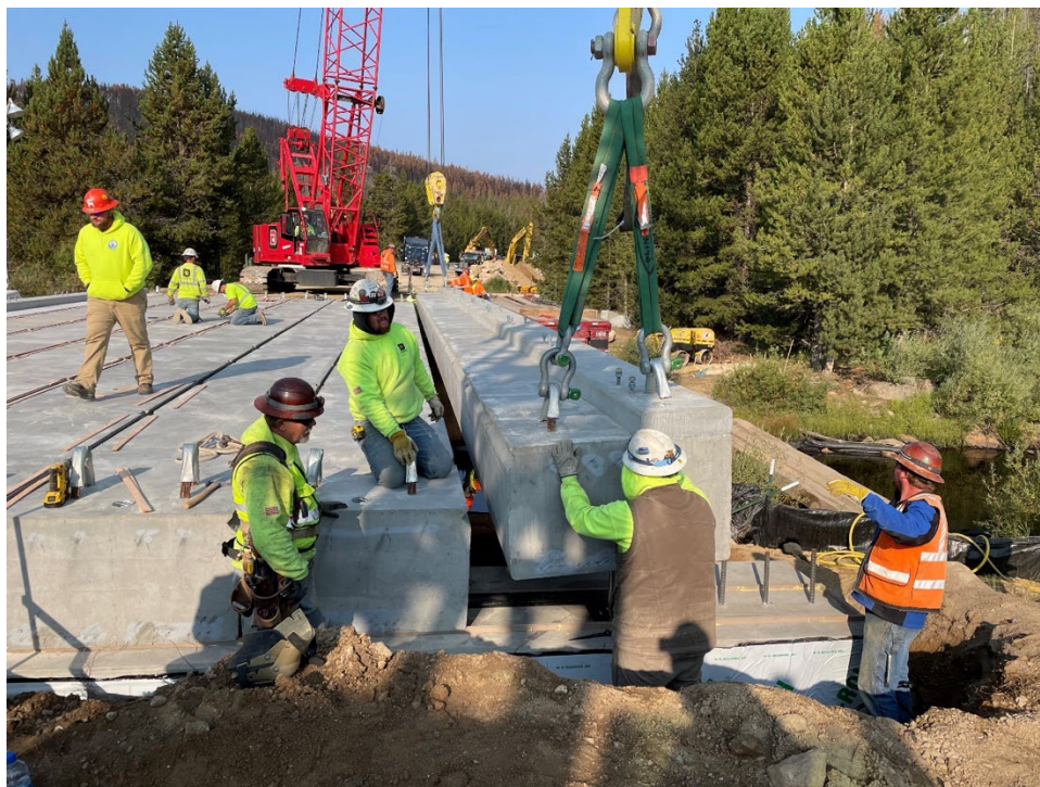
Figure 54: Final longitudinal deck element being placed
