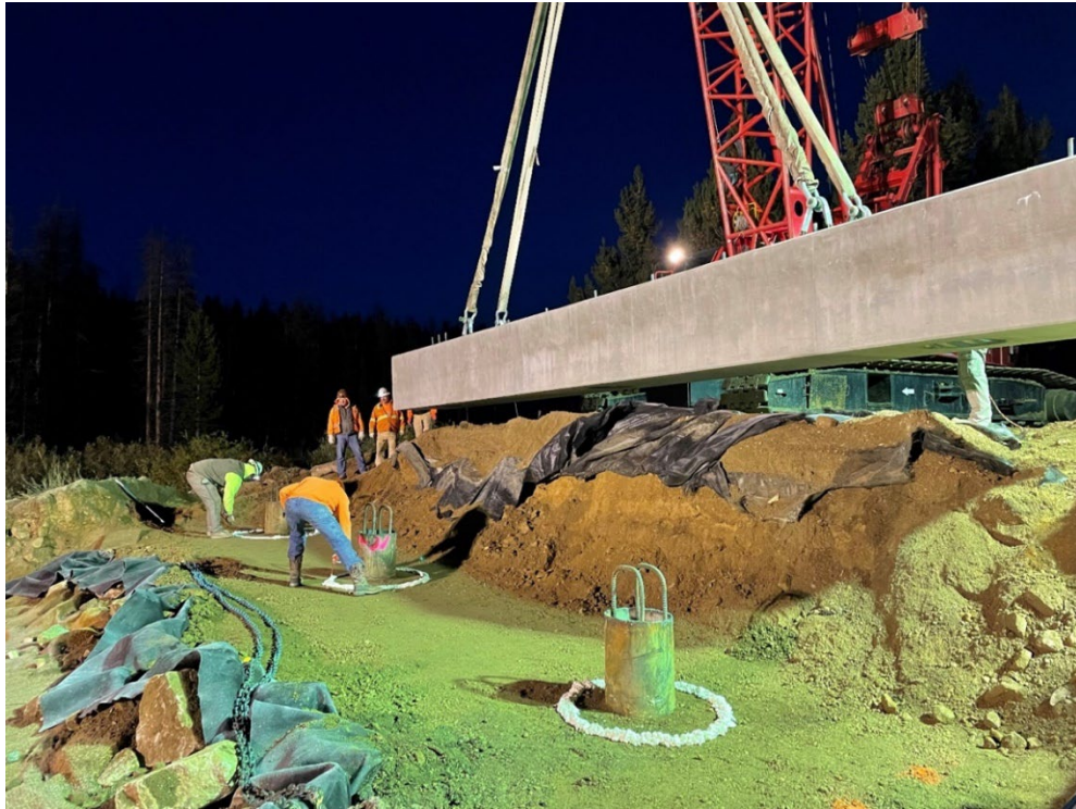
Figure 43: Uncovered pile caps and prepared surface prior to cap placement
