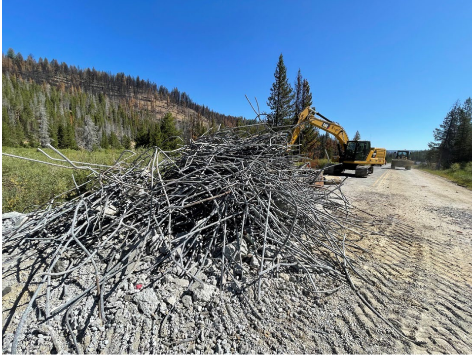
Figure 42: Reclaimed rebar from demolished bridge
