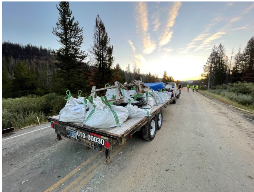
Figure 24: Sacks of MT-UHPC dry material on the jobsite
