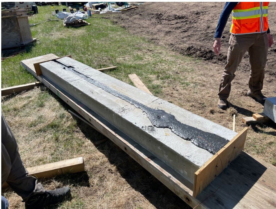
Figure 36: Sloped keyway mockup after MT-UHPC placement
