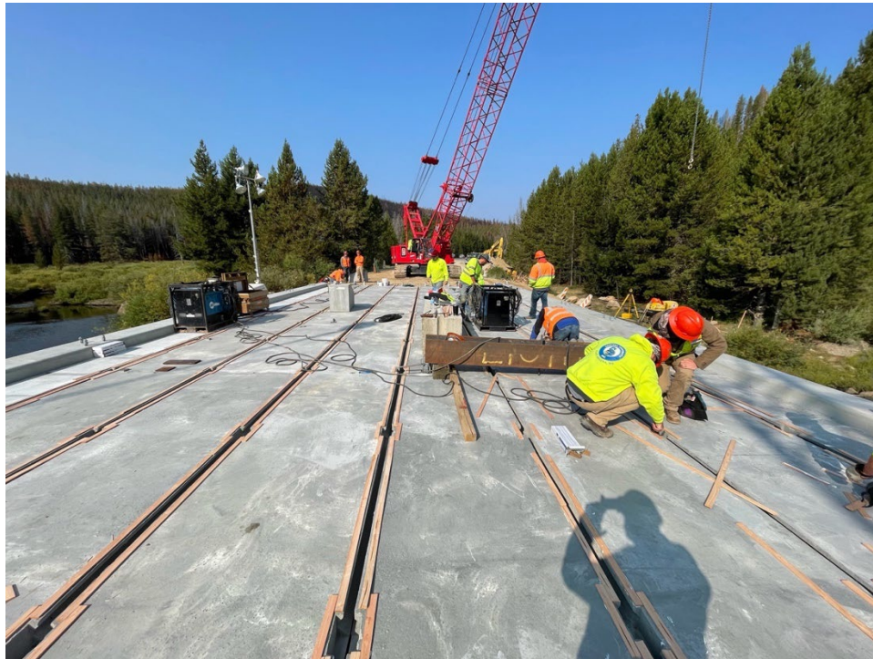
Figure 57: Wood slats glued to the top surface of beams around keyways
