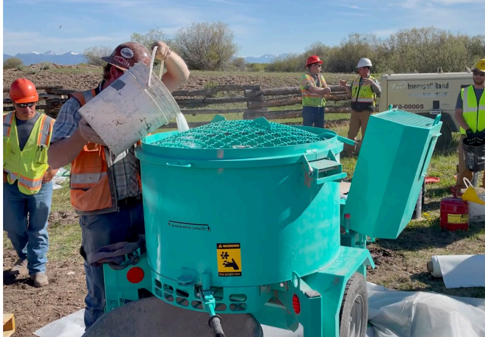
Figure 31: Water and HRWR being added to mixer
