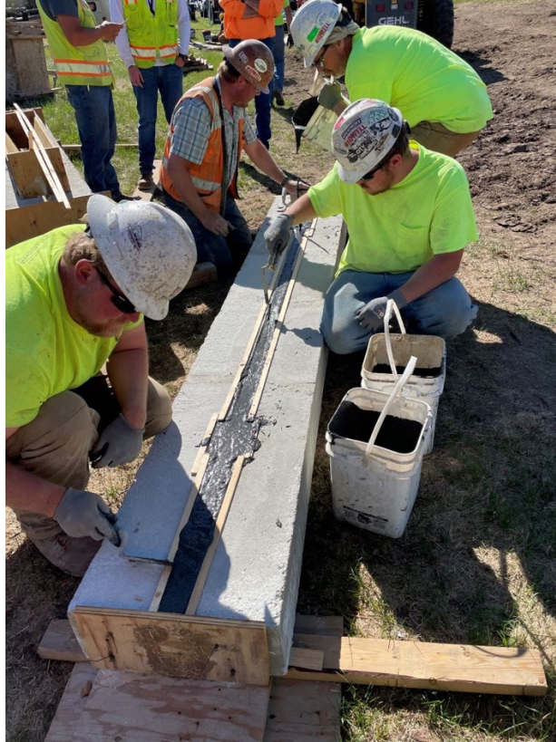
Figure 35: Flat keyway mockup after MT-UHPC placement
