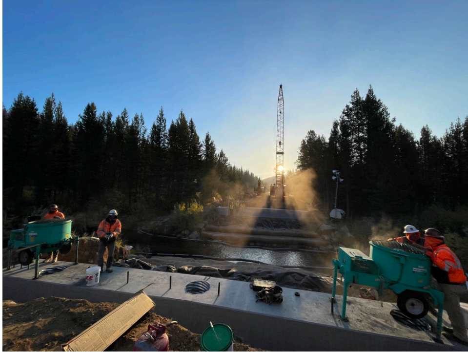
Figure 47: MT-UHPC placement on pile cap
