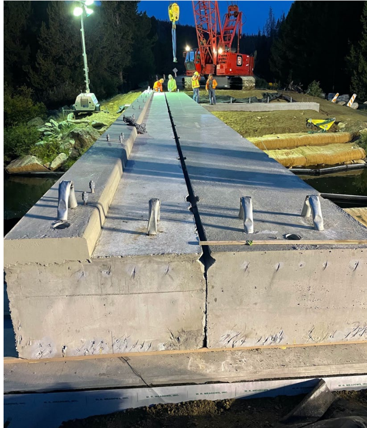
Figure 53: First two beam elements after placement, with visible keyway
