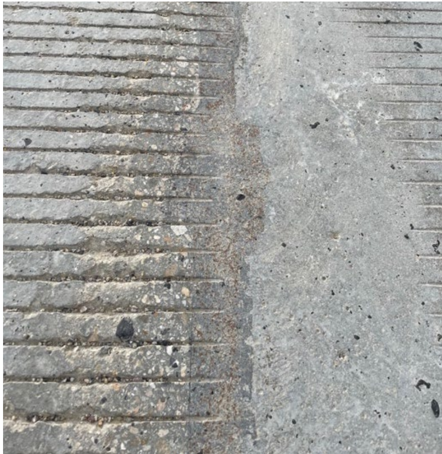
Figure 73: Another closeup of keyway joint from east bridge
