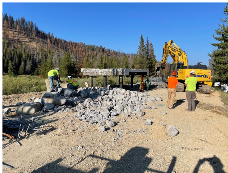
Figure 41: Demolished bridge after removal
