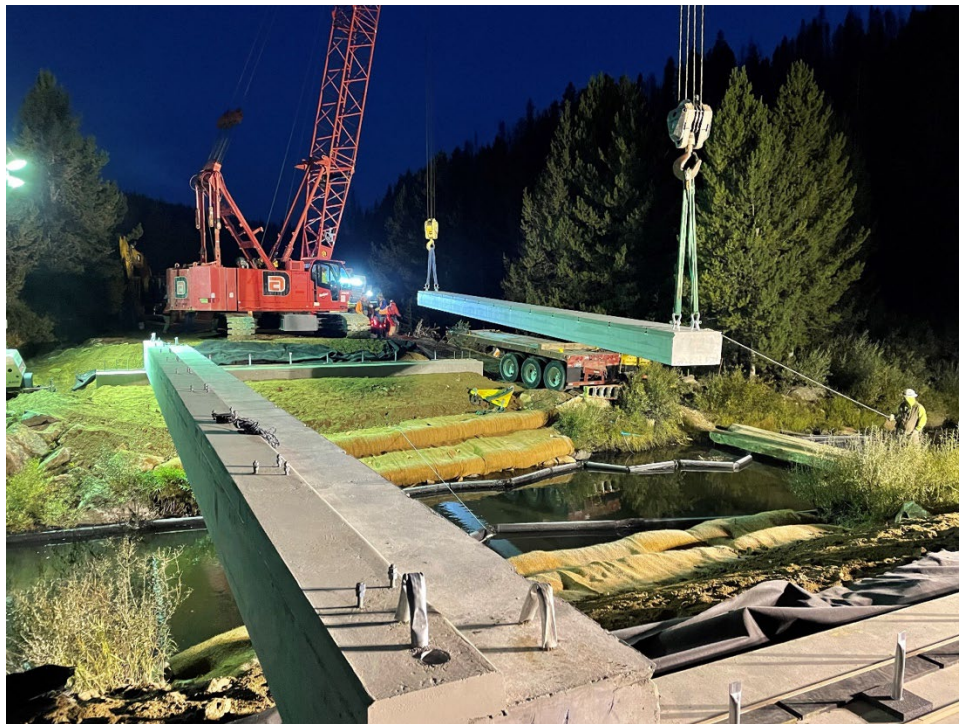
Figure 52: Second beam element being placed on pile caps
