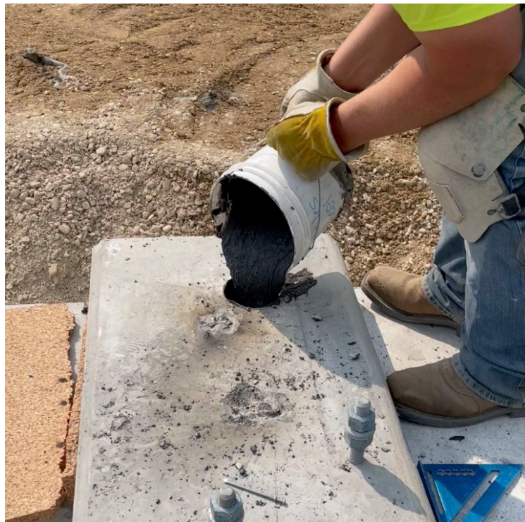
Figure 59: UHPC being placed into beam dowel hole, connecting it to pile cap
