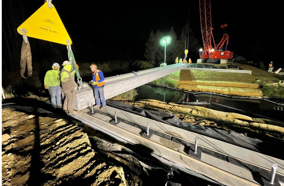
Figure 51: First longitudinal beam element being placed
