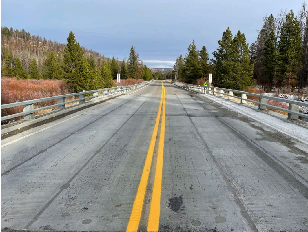
Figure 74: Overview of west bridge
