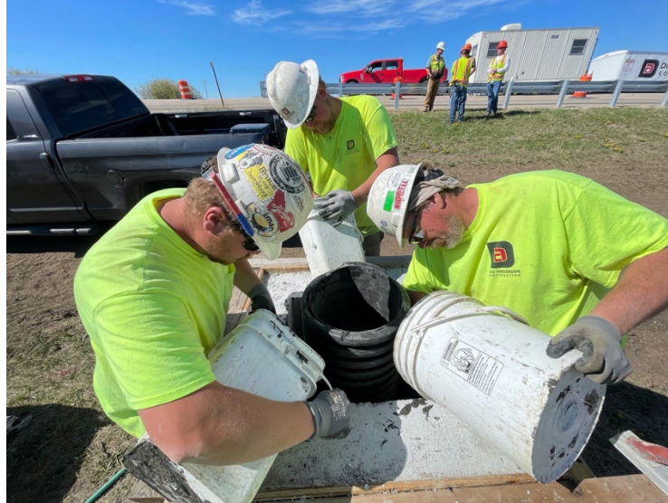
Figure 39: UHPC being added to the pile cap connection mockup
