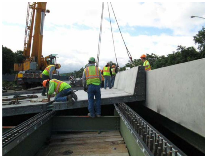
Figure 5: Example precast UHPC project in progress
