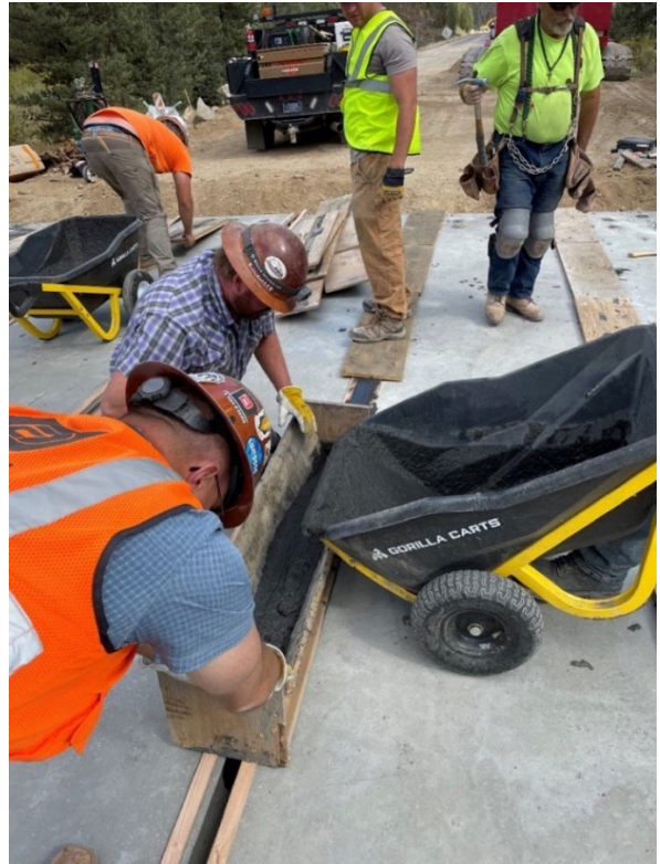
b) UHPC being added to keyway using trough
