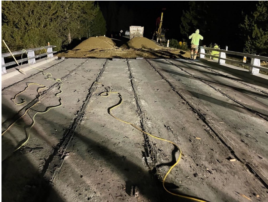
Figure 62: Keyways after removal of wood slats, just prior to grinding
