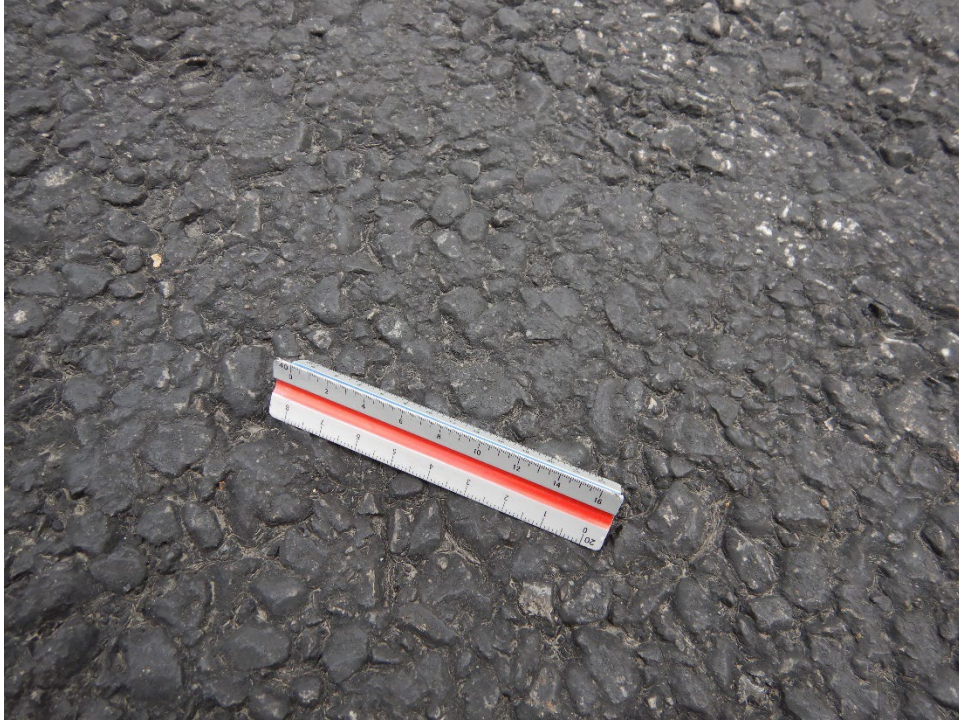
Figure UDOT-35. BMC Taxiway (Rehabilitated in 2006) Surface Texture
