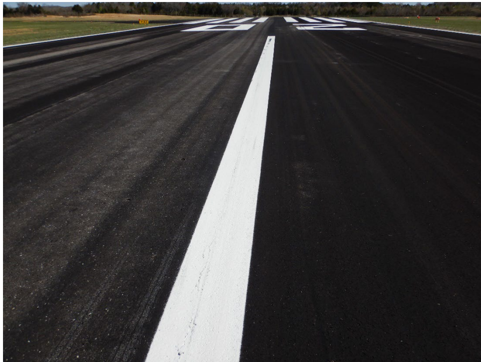
Figure LUG-3. P-608 Coverage on Runway 02/20
