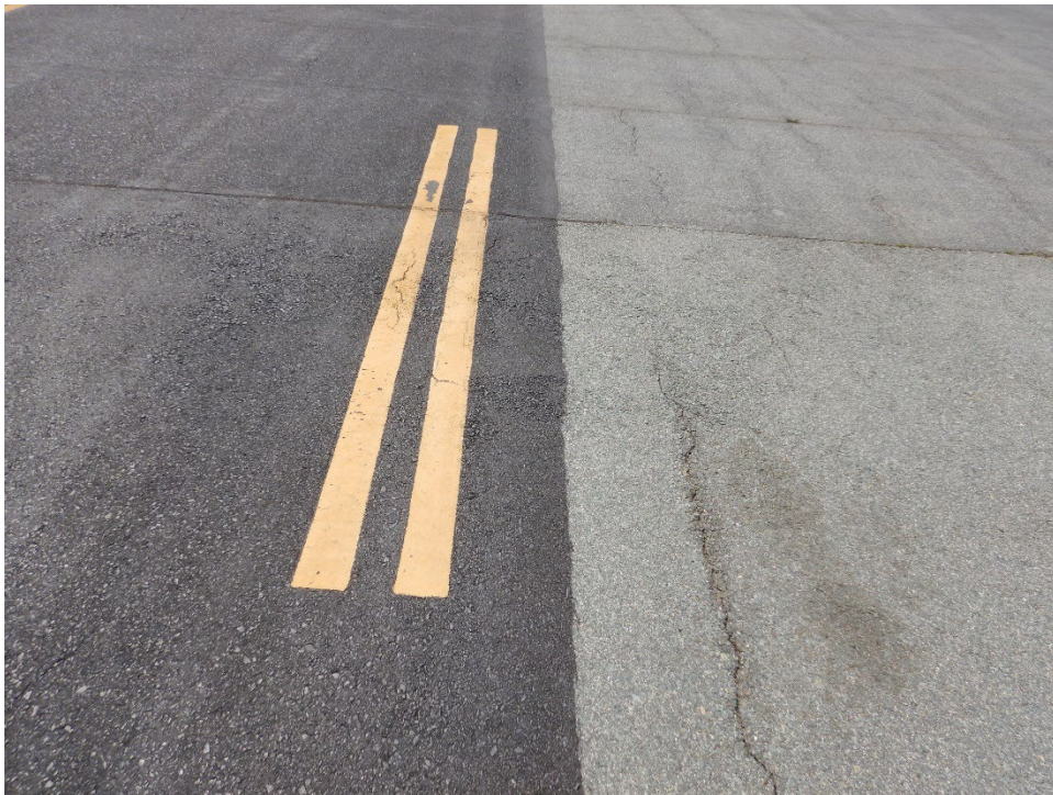
Figure EQY-19. Overview of Edge of P-632 Application on High Age Taxiway
