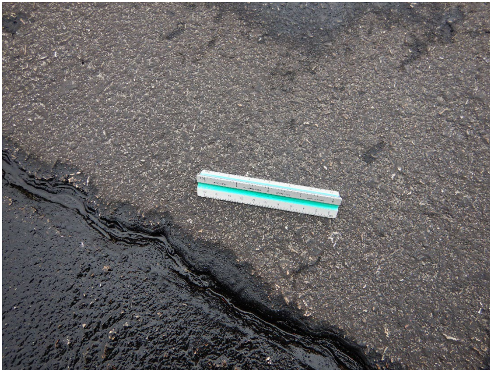
Figure EKO-31. Crack Sealant Condition on Taxiway B
