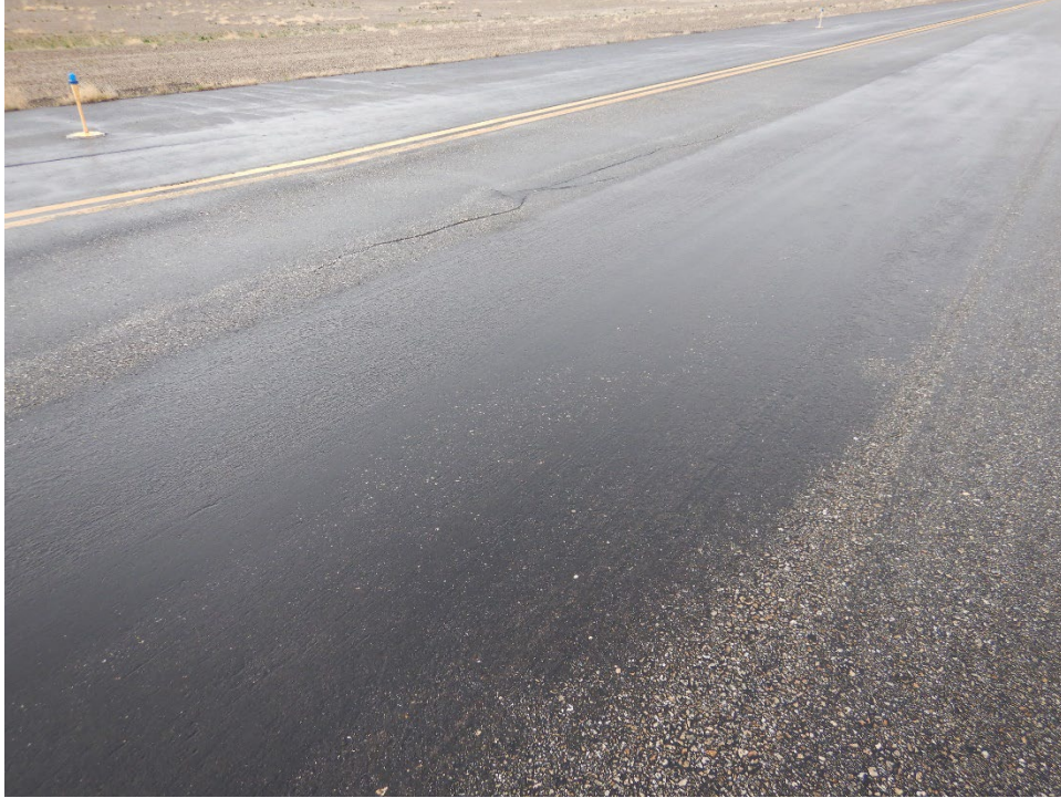
Figure EKO-10. Thicker P-608 Application on Taxiway A
