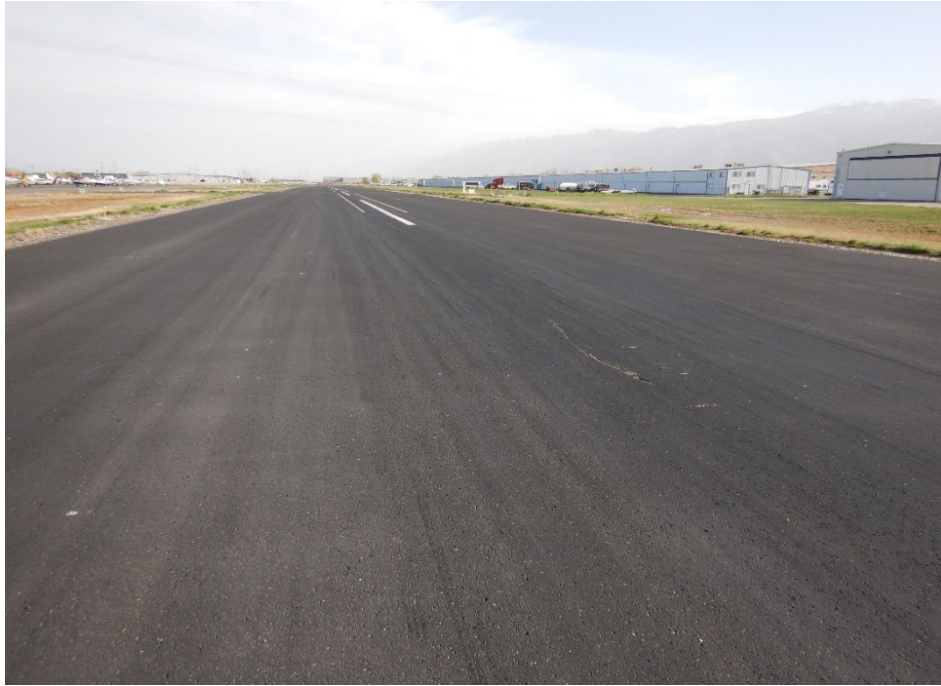
Figure UDOT-3. Overview of BTF Runway 17/35 With Onyx
