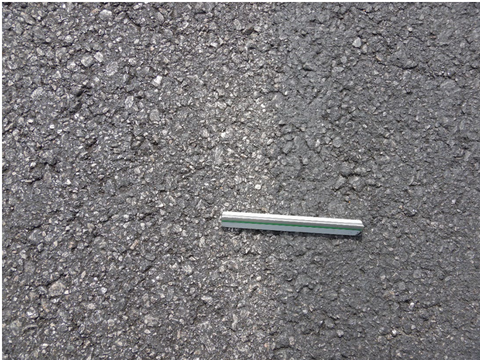
Figure EQY-13. Medium Age Taxiway Without (Left) and With (Right) P-632
