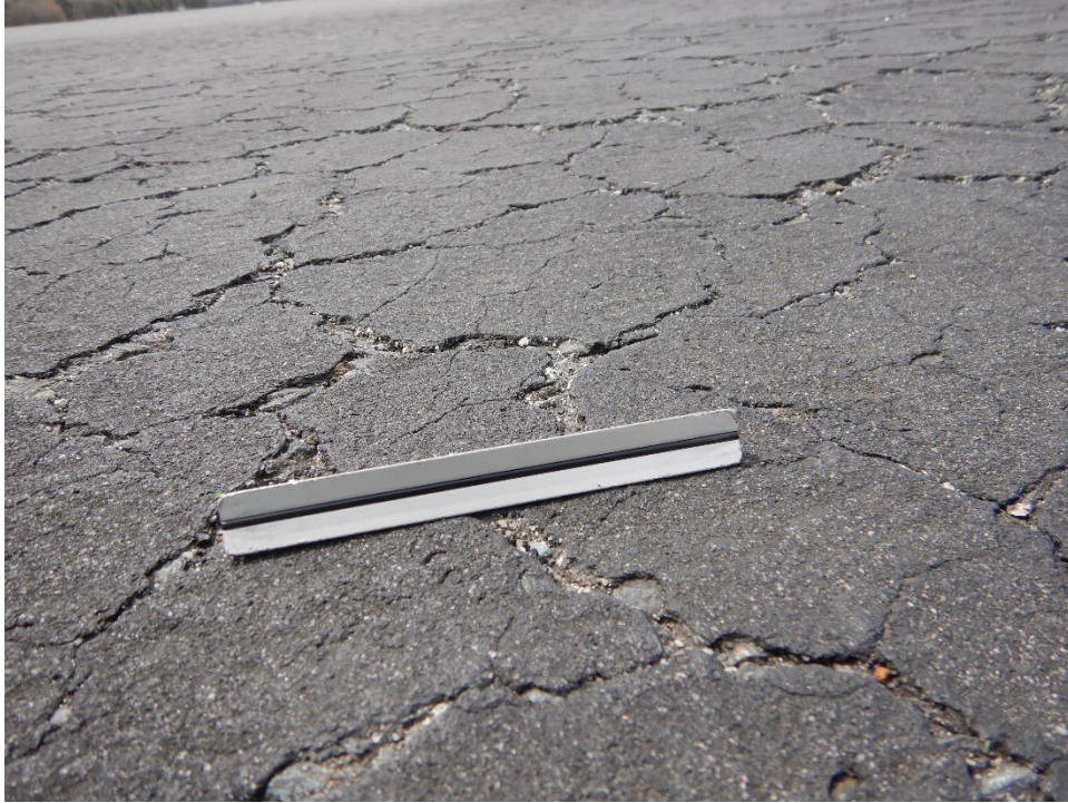
Figure EQY-3. Coal Tar Slurry Texture
