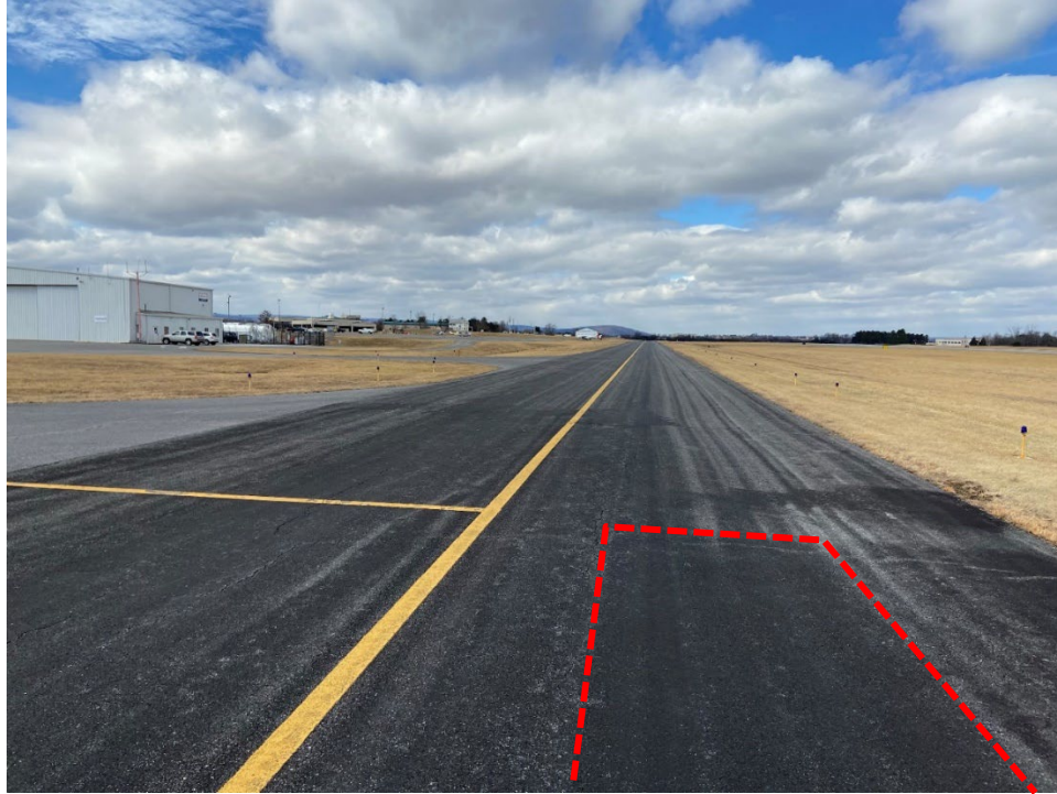
Figure 8. Typical P-608 Application and Overlap on Taxiway A
