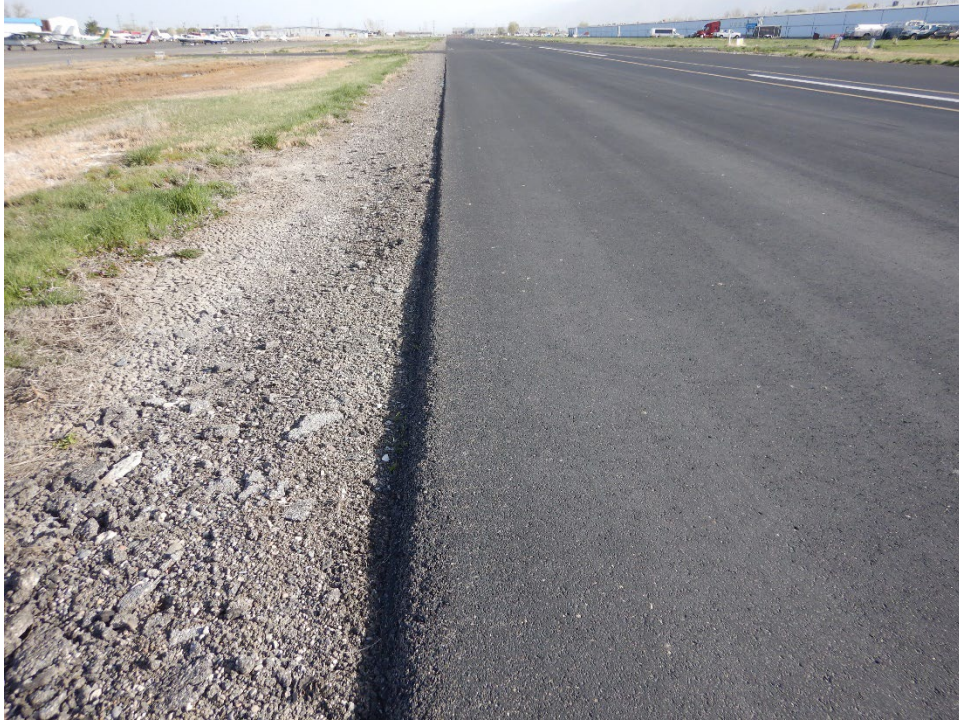
Figure UDOT-7. Overview of Edge of BTF Runway 17/35 With Onyx
