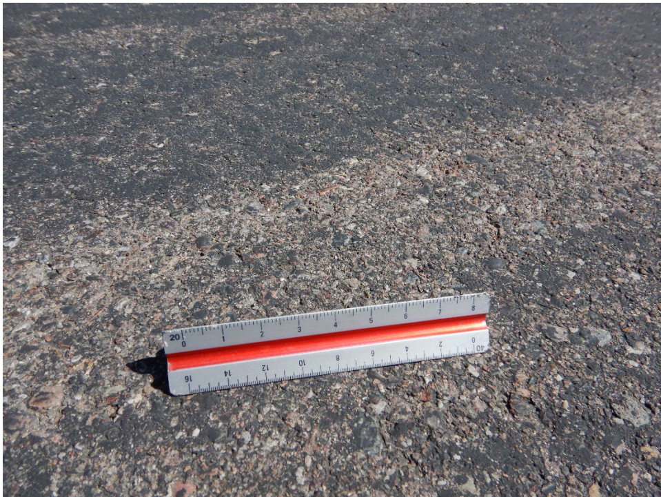
Figure PHX-11. East Cargo Apron Texture
