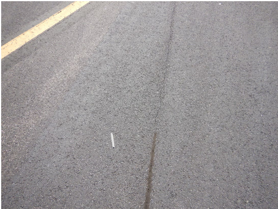
Figure EQY-15. Longitudinal Paving Joint on Medium Age Taxiway
