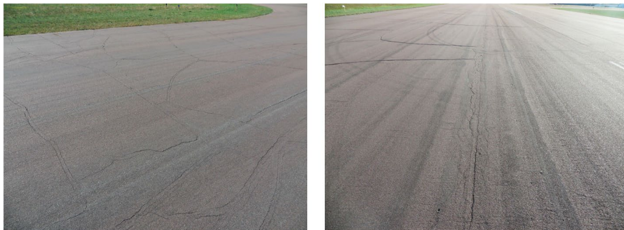
Figure WisDOT-1. P-626 (left) and WisDOT P-652 (right) at STE (September 2017)
