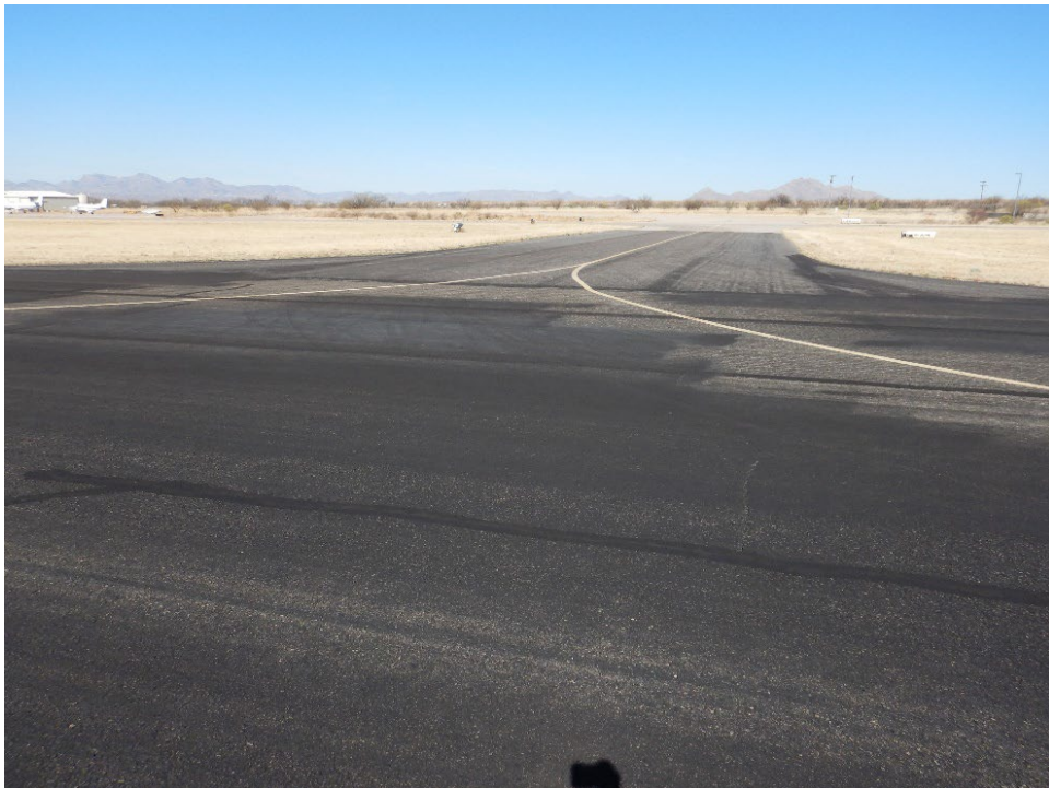
Figure OLS-3. P-608 Coverage on Runway 04/22 and Connector
