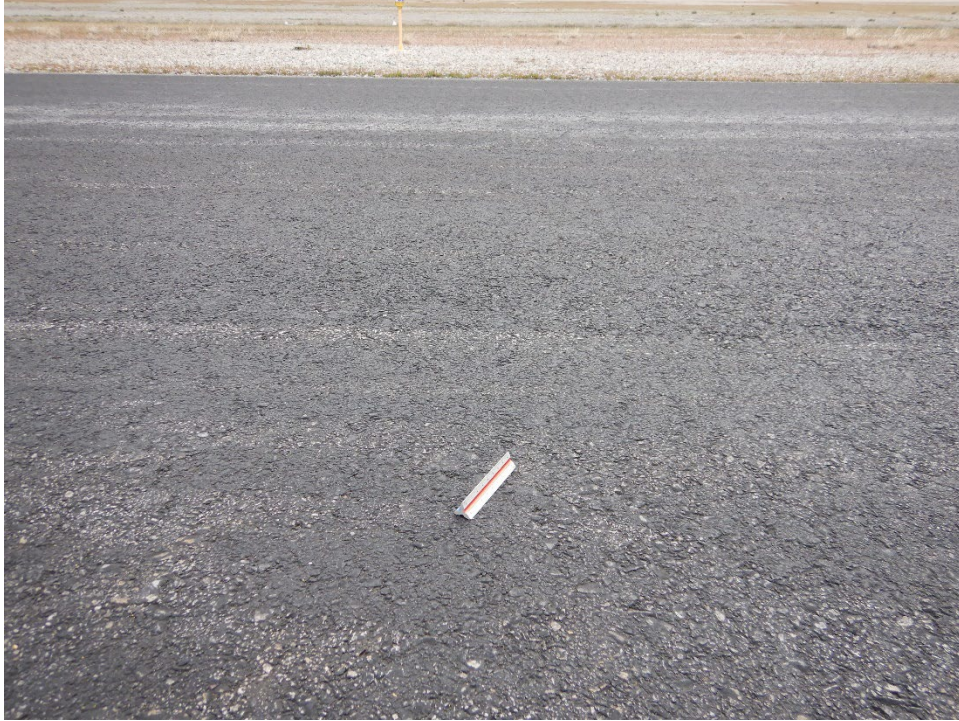
Figure UDOT-29. Closeup of BMC Taxiway (Rehabilitated in 2008) Surface
