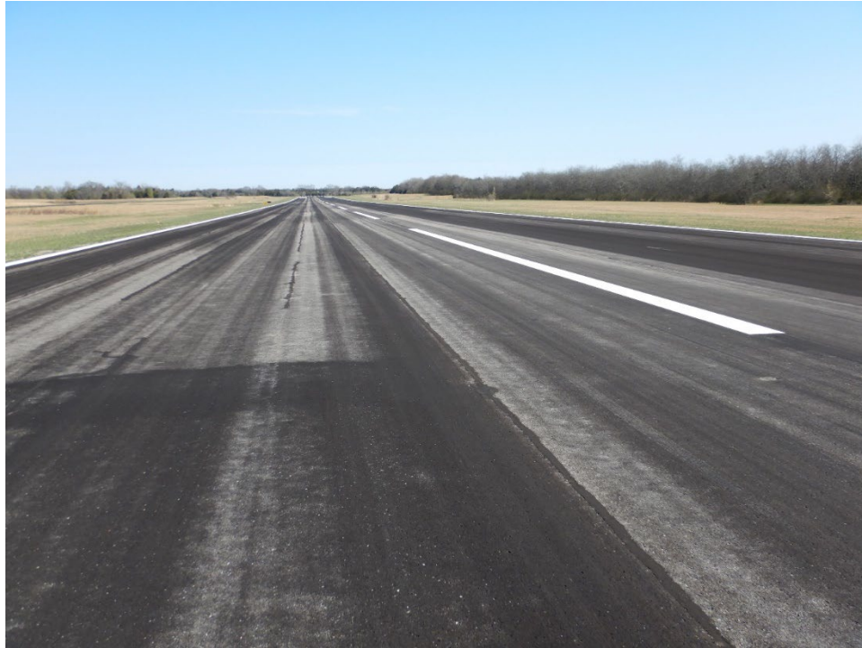
Figure 11. Ellington Airport Runway 02/20
