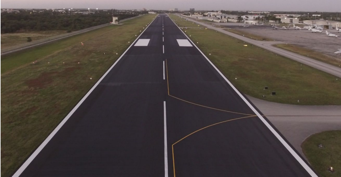
Figure BCT-1. Runway 05/23 Shortly After P-608-R Application
