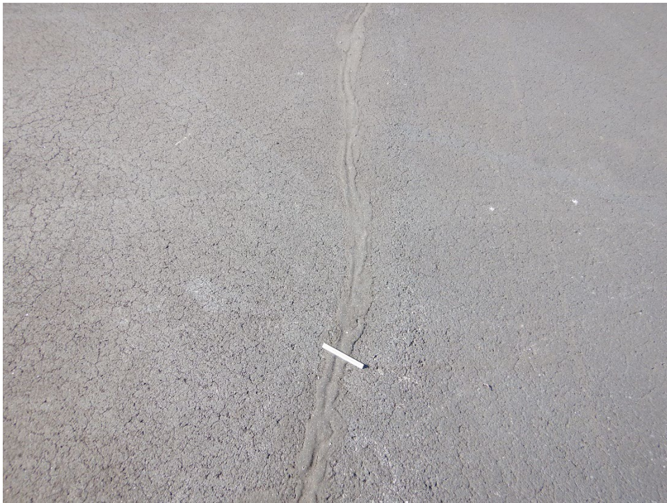
Figure LUG-16. Crack Sealant on Apron
