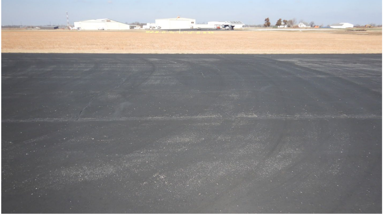
Figure MoDOT-21. MO-623 Application Pattern at LLU
