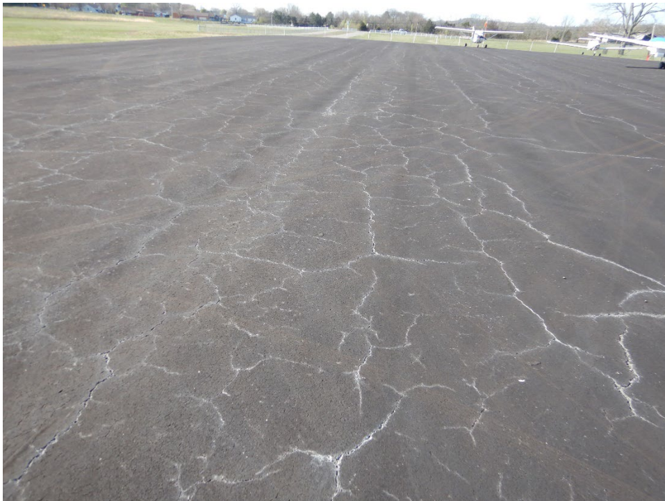
Figure LUG-12. Apron Overview With P-608 With White Precipitate
