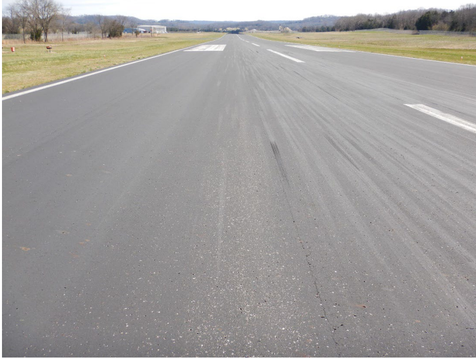
Figure GZS-4. Tire Marks on Runway 16/34
