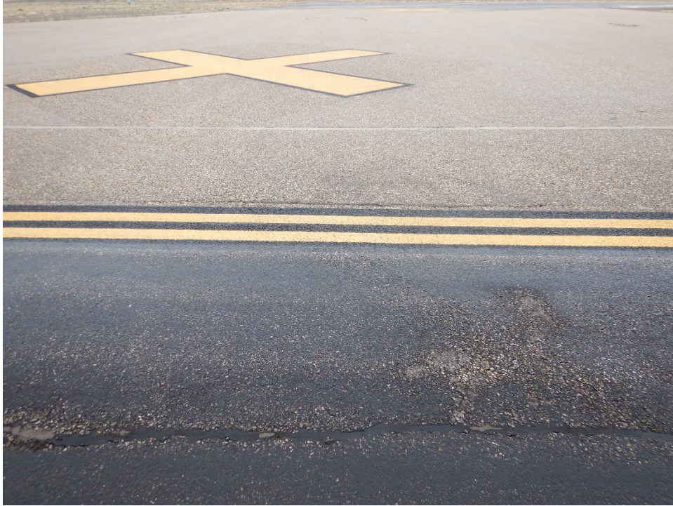
Figure EKO-18. P-608 Treated and Untreated Areas
