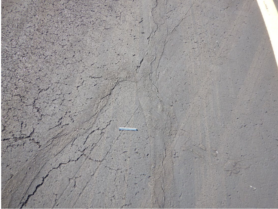
Figure LUG-22. Crack Sealant on Taxiway A in High-Age Area
