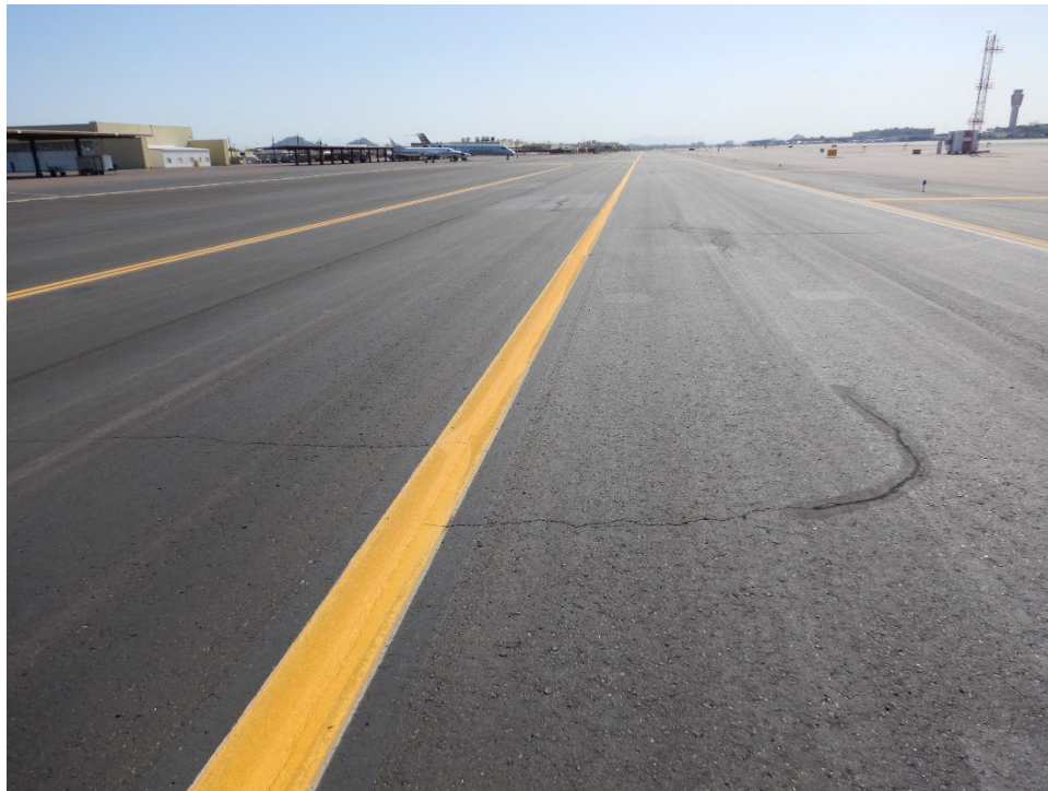
Figure PHX-5. Overview of Taxiway A With Acrylic Coat (East Facing)
