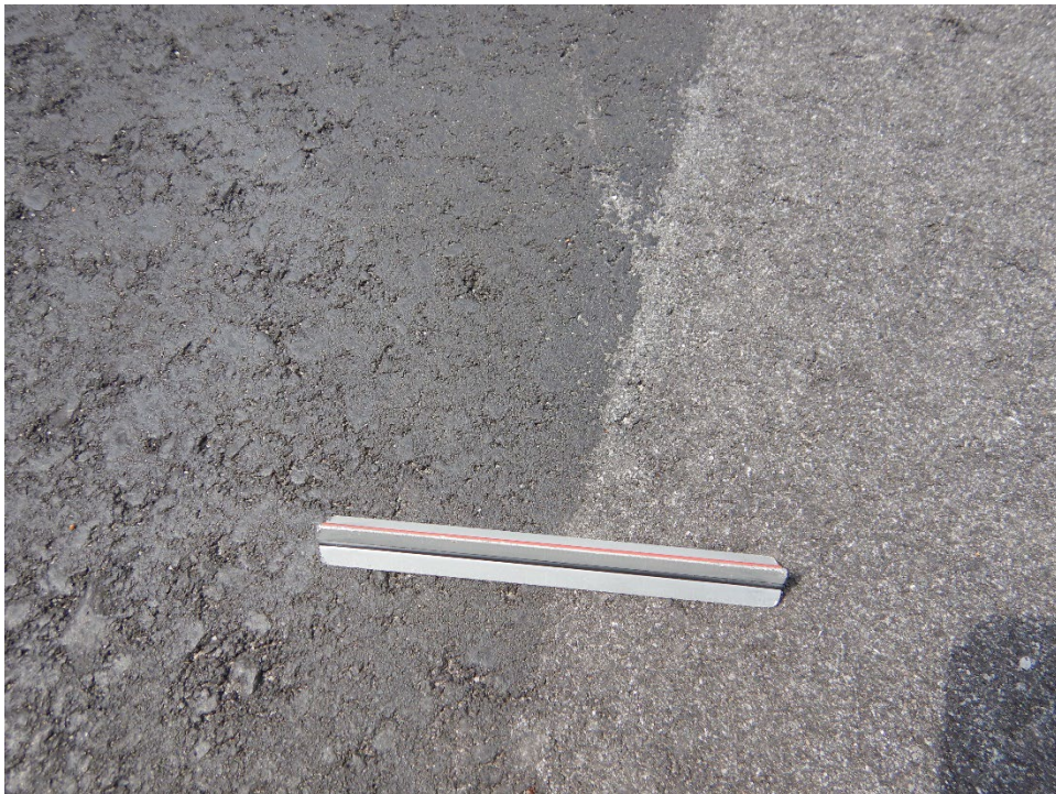
Figure EQY-7. Apron with (Left) and Without (Right) P-631
