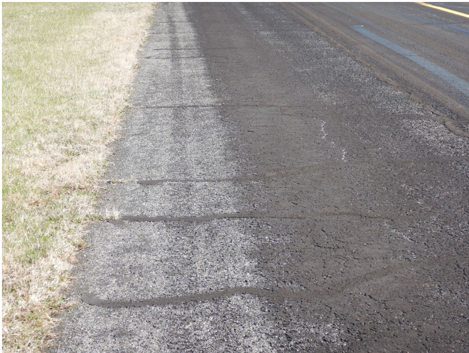
Figure LUG-23. P-608 Coverage on Taxiway A Edge in High-Age Area
