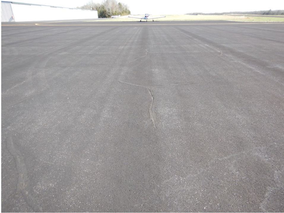
Figure LUG-11. Overview of Apron With P-608
