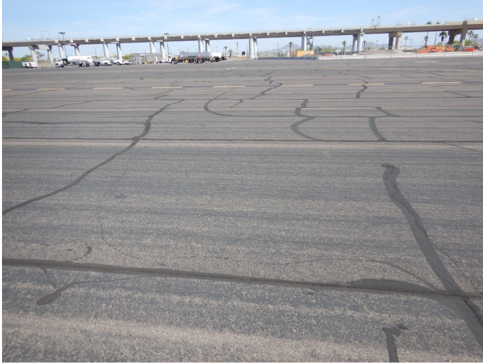
Figure PHX-10. East Cargo Apron Overview With Acrylic Coat
