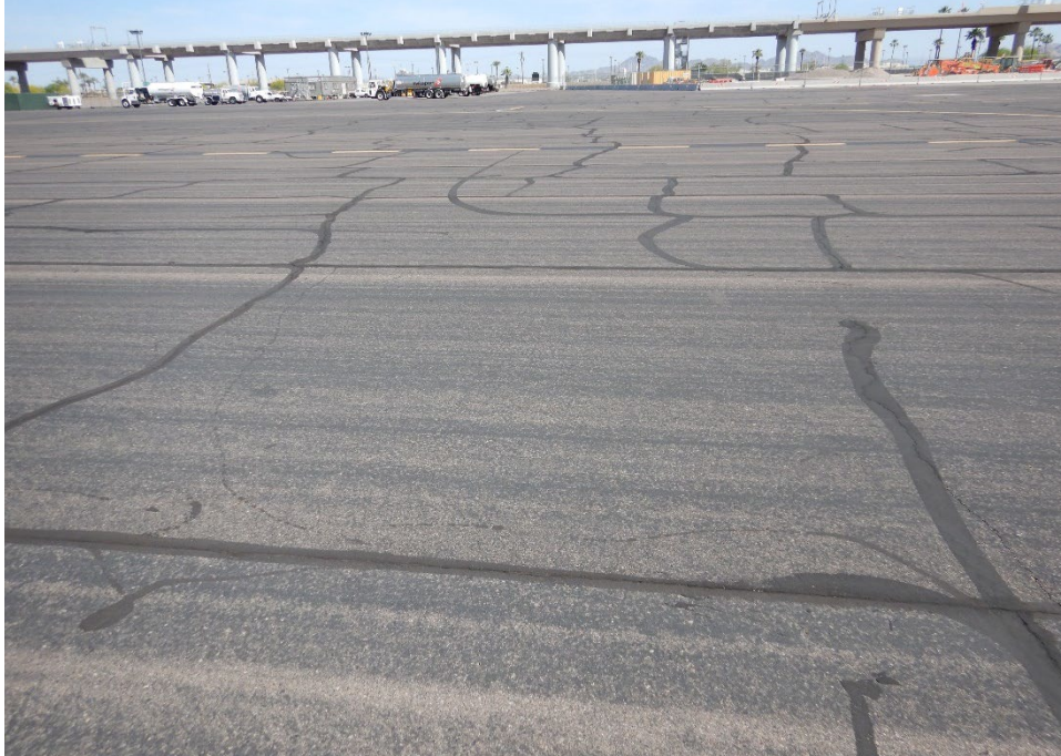
Figure 7. East Cargo Apron at PHX With Acrylic Coat
