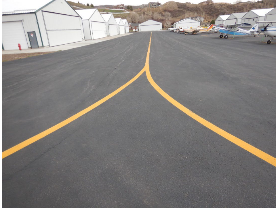
Figure UDOT-27. Overview of 42U Apron With Onyx
