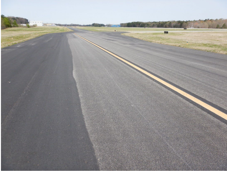
Figure EQY-12. Overview of P-632 Coverage on Medium Age Taxiway
