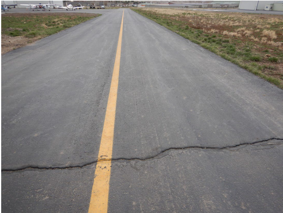
Figure UDOT-24. Overview of 42U Taxiway With Onyx
