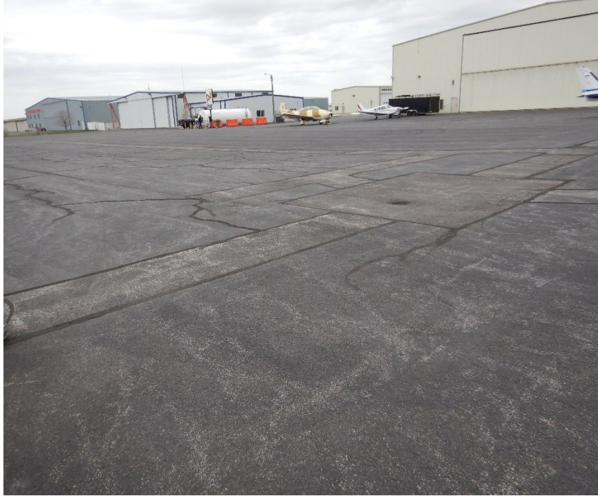
Figure UDOT-40. Overview of BMC Apron With Coal Tar Fog Seal
