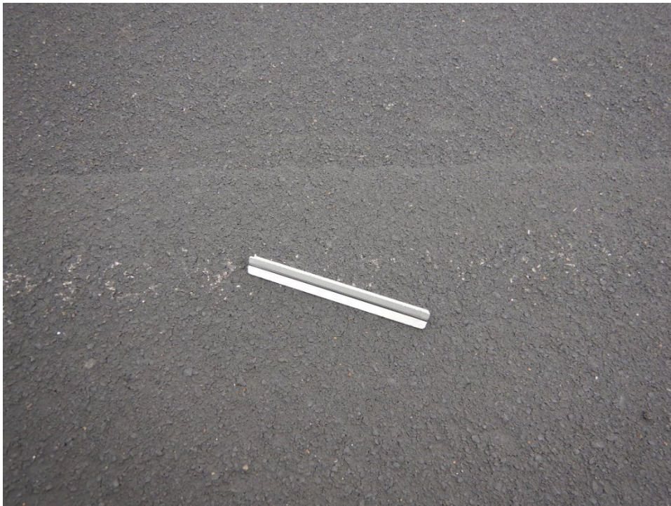
Figure MoDOT-4. P-629 Texture on M17 Taxiway
