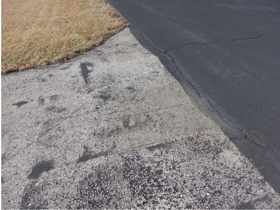
Figure MoDOT-17. Untreated Pavement (Left) and Pavement Treated With MO-623
