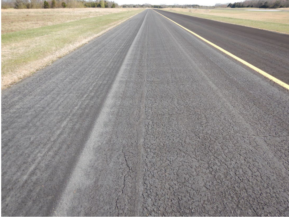
Figure LUG-25. Taxiway A With P-608H
