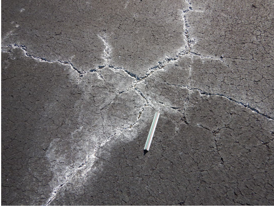
Figure LUG-17. Closeup of White Precipitate on Apron
