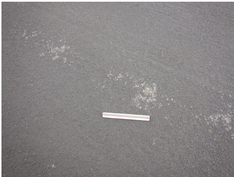
Figure MoDOT-2. P-629 Texture on M17 Runway 18/36
