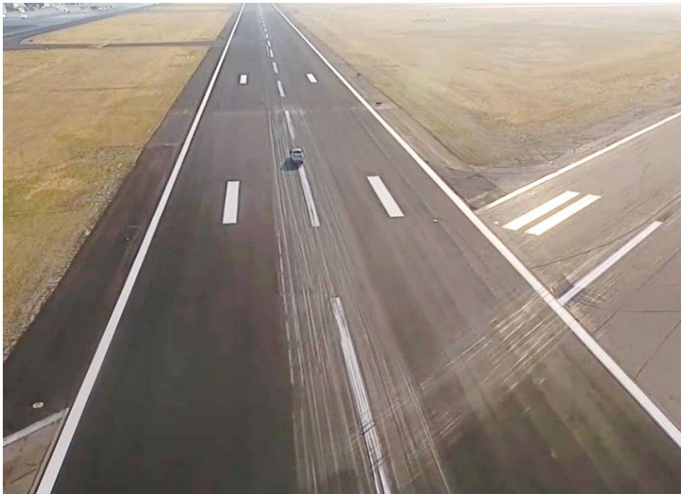
Figure WYDOT-3. Drone View of P-608-R Shortly After Initial Application—October 2020
