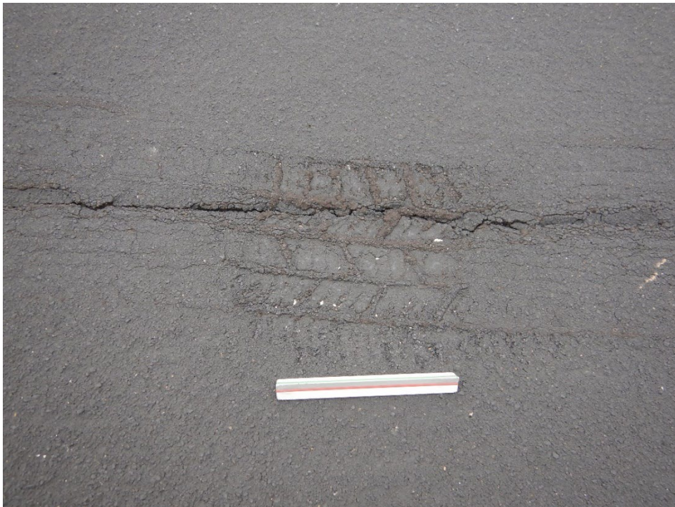
Figure MoDOT-8. Tire Imprint on P-629
