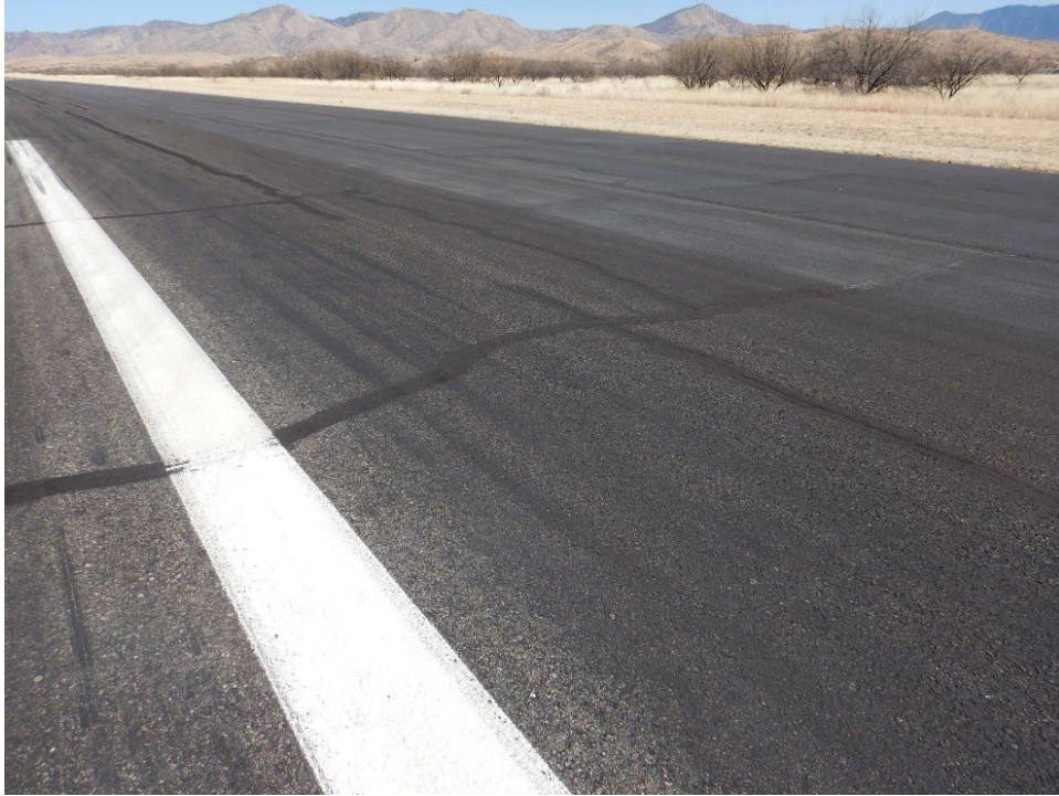
Figure OLS-2. Wearing Pattern on Runway 04/22
