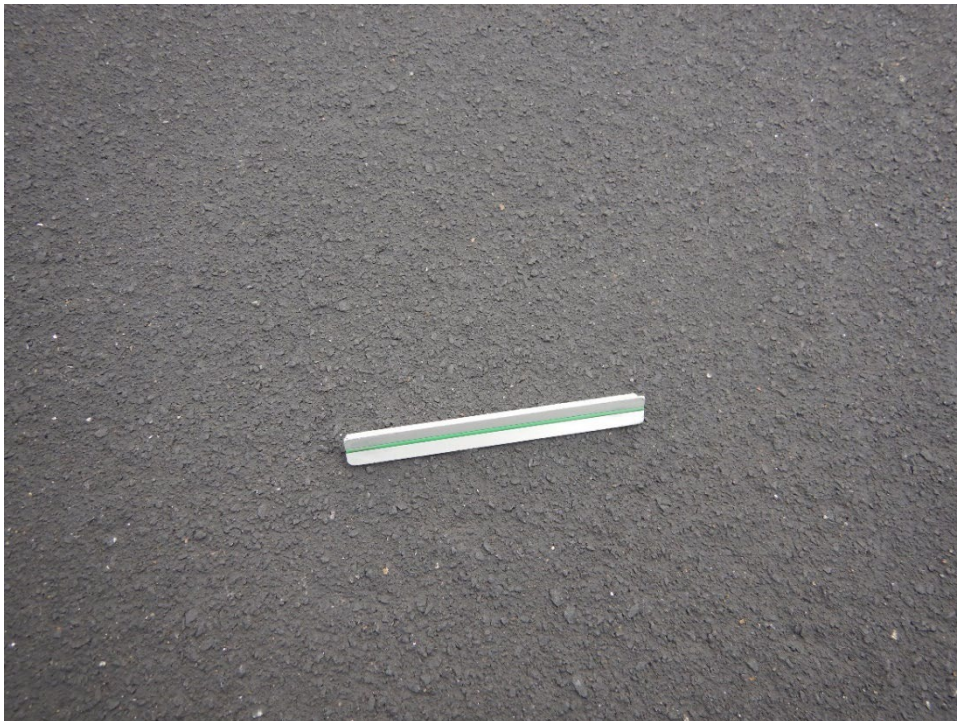
Figure MoDOT-6. P-629 Texture on M17 Apron
