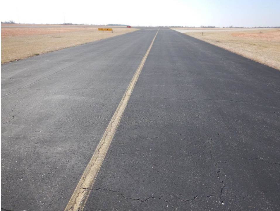
Figure MoDOT-13. Overview of LLU Taxiway With MO-623
