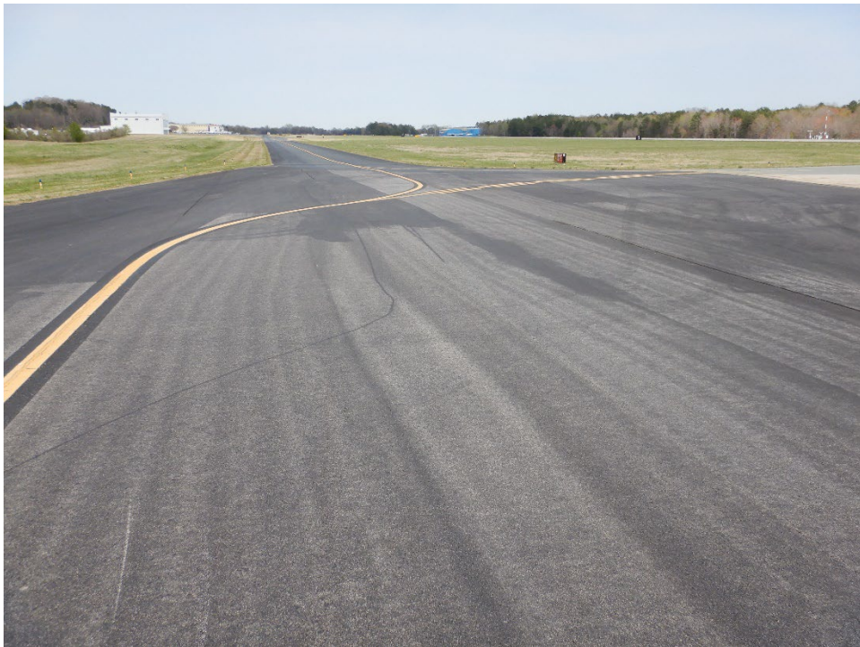
Figure EQY-11. Overview of P-632 Coverage on Medium Age Taxiway
