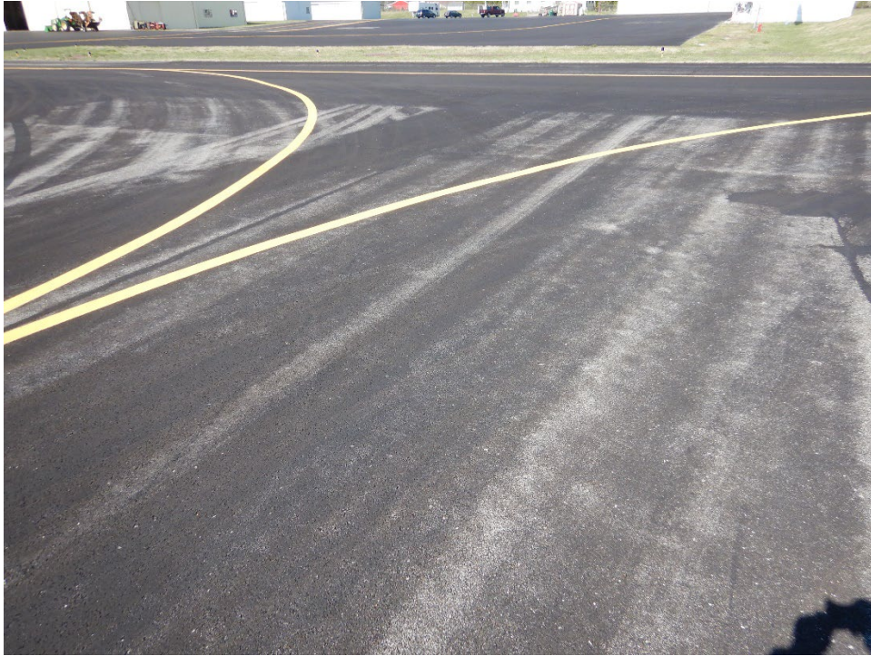
Figure LUG-6. Overview of Taxiway A1 With P-608
