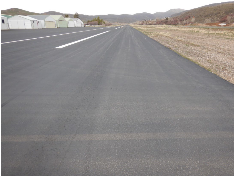
Figure UDOT-18. Overview of 42U Runway 03/21 With Onyx
