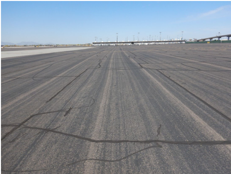
Figure PHX-9. East Cargo Apron Overview With Acrylic Coat
