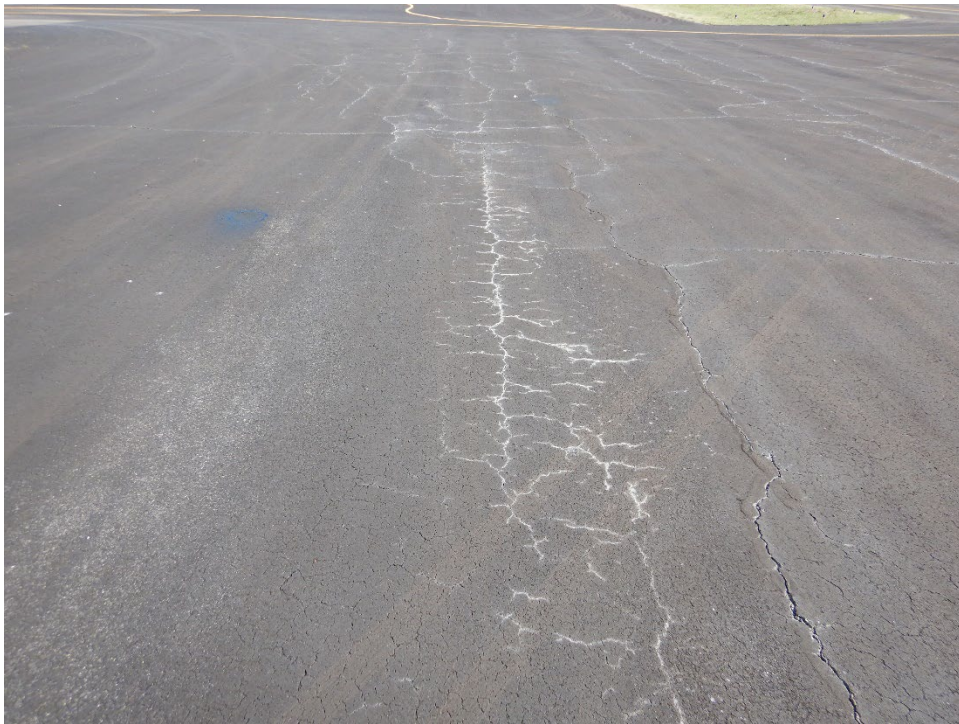
Figure LUG-18. Overview of White Precipitate on Apron
