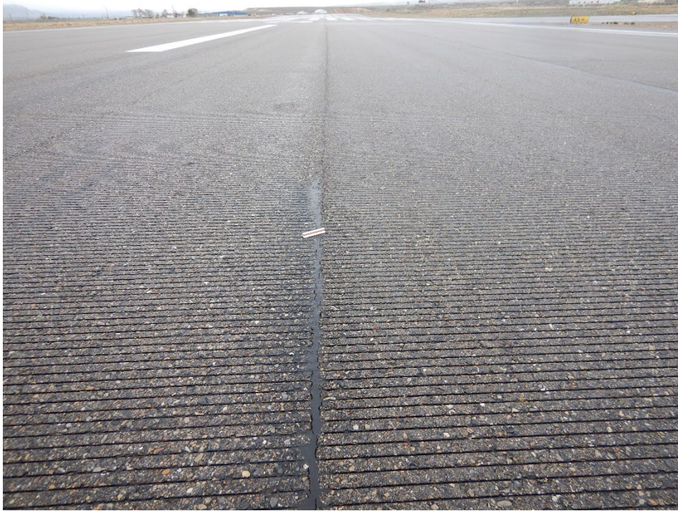
Figure EKO-5. Sealed Longitudinal Paving Joint on Runway 06/24
