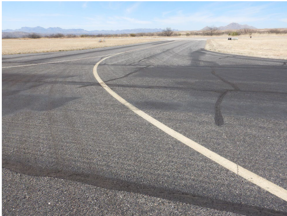
Figure 6. P-608 Coverage Along Taxi Line at OLS
