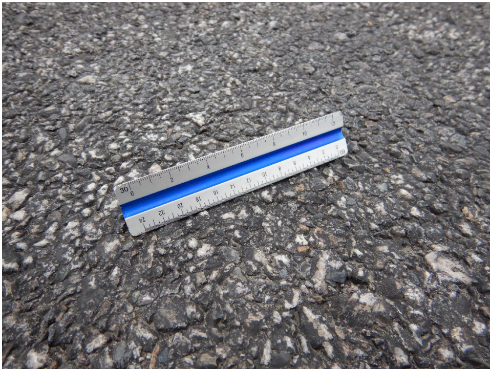
Figure UDOT-41. BMC Apron Surface Texture
