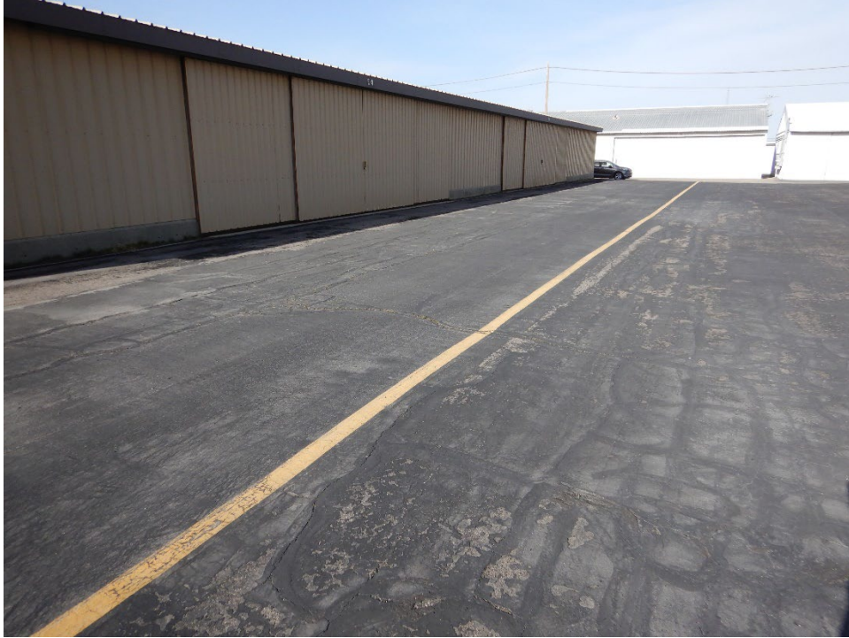
Figure UDOT-13. Overview of BTF Apron With Onyx
