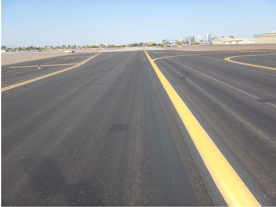
Figure PHX-6. Overview of Taxiway A With Acrylic Coat (West Facing)
