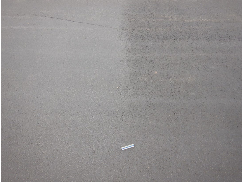
Figure UDOT-23. Onyx Color Difference Due to Application Phase Break
