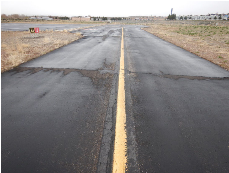
Figure EKO-27. Taxiway B Overview
