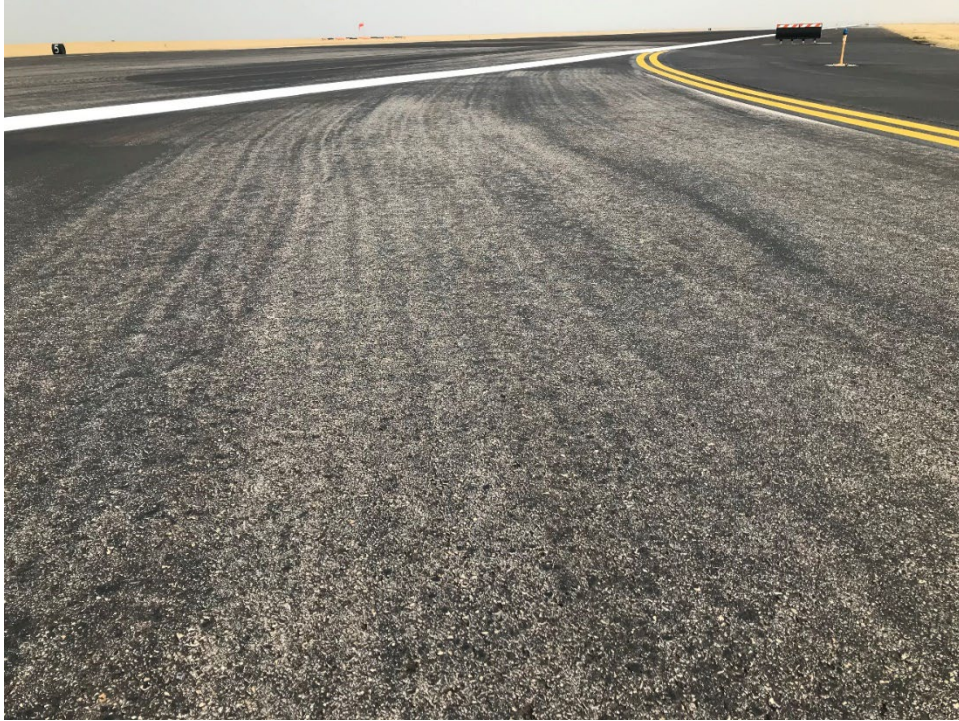
Figure WYDOT-2. P-608-R Shortly After Initial Application—September 2020
