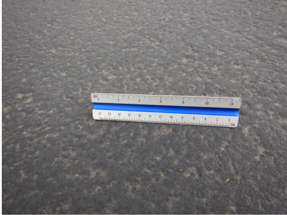
Figure UDOT-19. Surface Texture of 42U Runway 03/21
