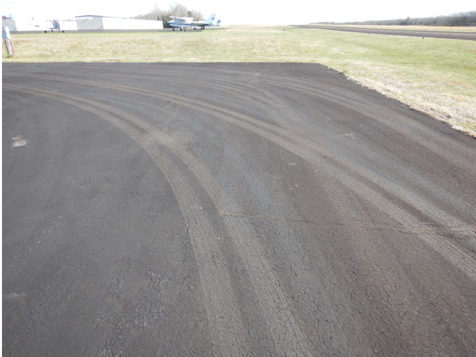
Figure LUG-14. Fuel Truck Track on P-608 Over P-631
