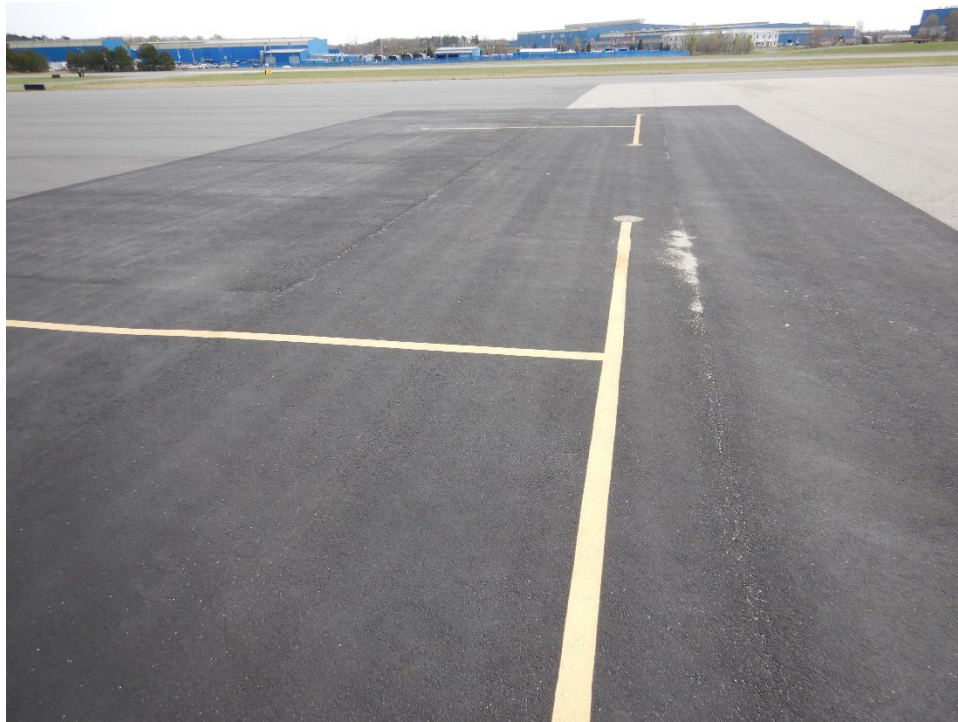
Figure EQY-5. Apron Overview with P-631
