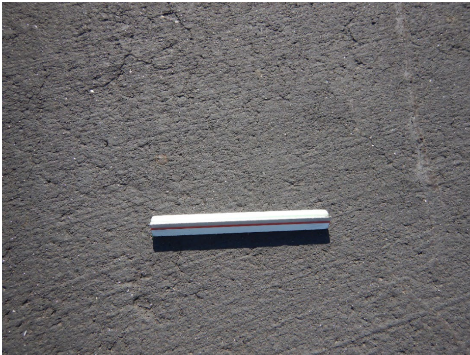
Figure MoDOT-12. MO-623 Texture on LLU Runway 03/21
