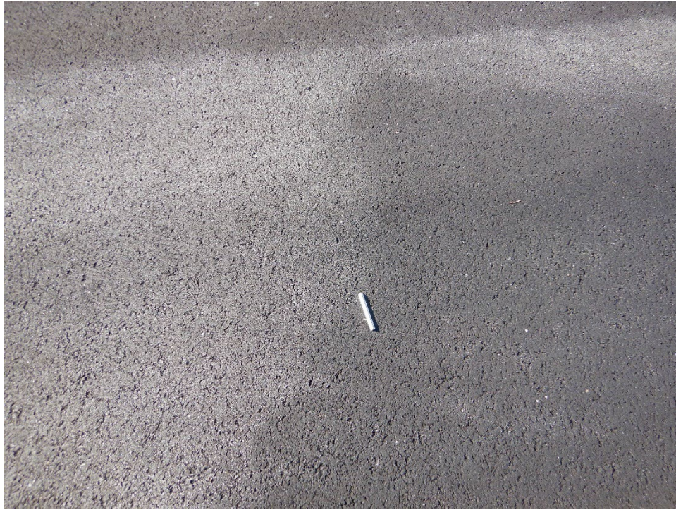
Figure LUG-10. Coverage on T-Hangar Pavement
