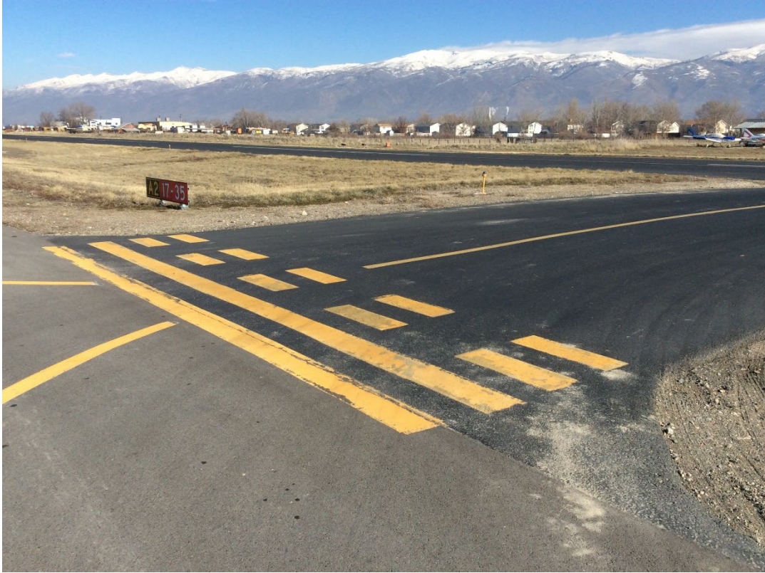
Figure UDOT-2. BTF Connector (right) With Onyx and Parallel Taxiway (Left) Without Onyx
