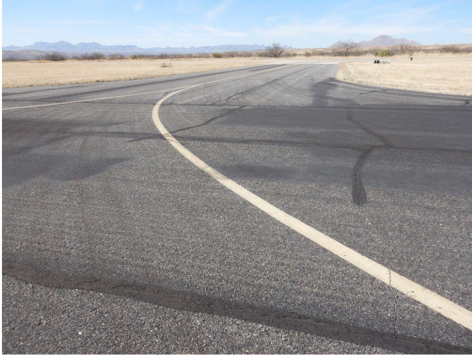
Figure OLS-4. P-608 Coverage on Connector
