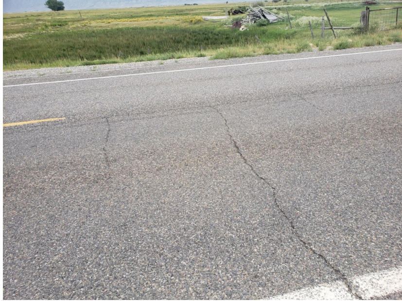
Figure 3.2 Section UT-03 showing thermal and reflective cracking
