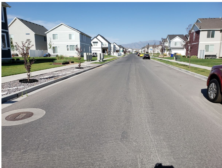
Figure 3.5 Section UT-07 showing no visible distresses
