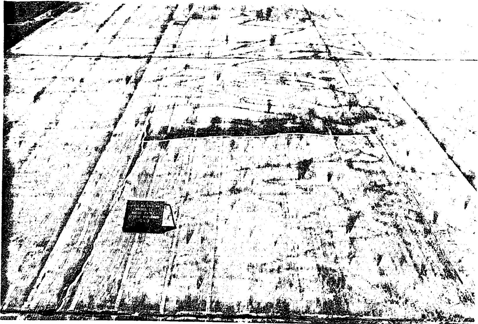
FIGURE 4-6. EXAMPLE OF A CONDITION FACTOR, "C r " OF 0.85 USED FOR CONCRETE OVERLAY DESIGN PURPOSES
