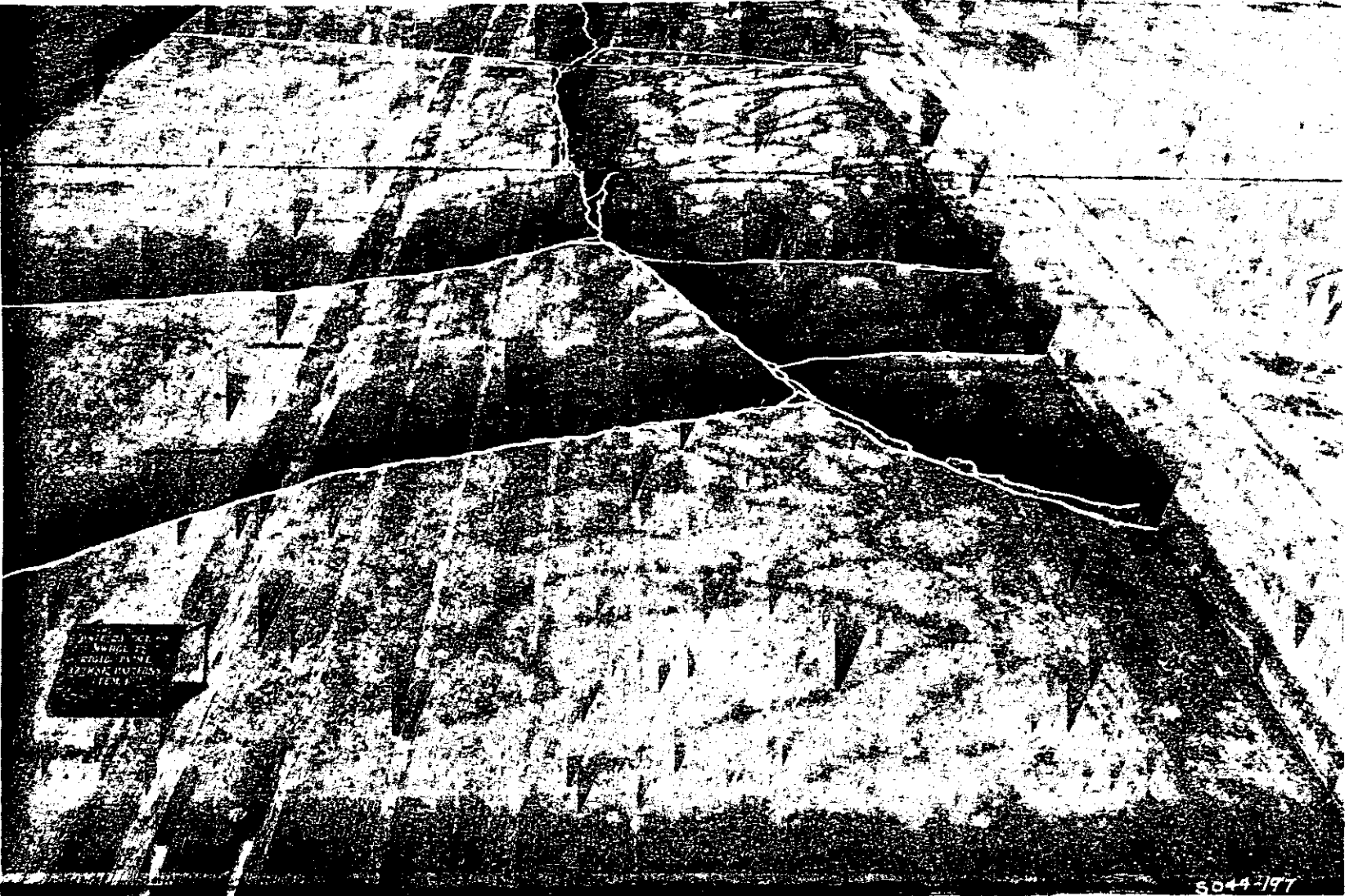
FIGURE 4-5. EXAMPLE OF A "C b " FACTOR OF 0.75 FOR BITUMINOUS OVERLAY DESIGN
