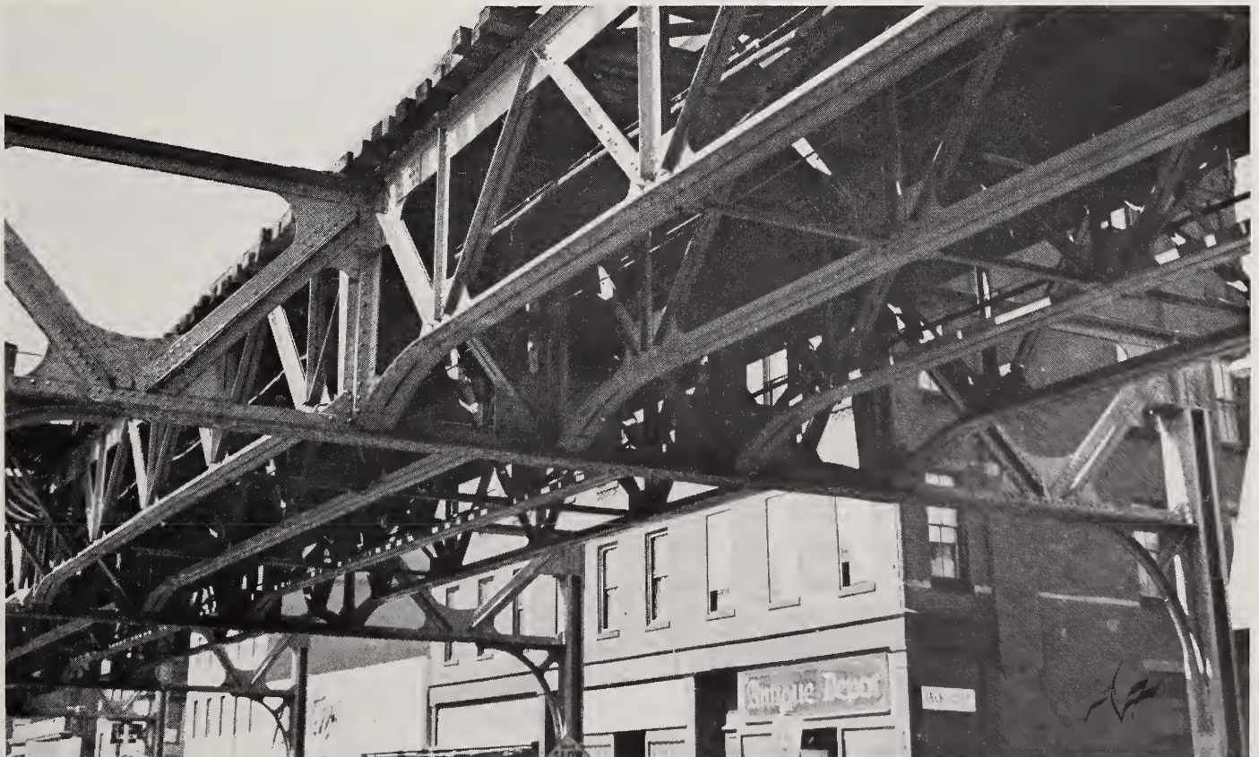
UMTA-sponsored research developed computer models to predict noise on three types of elevated structures — concrete deck on steel plate girder (left), open tie deck on steel plate girder (right), and open tie deck on open web girder (bottom).
