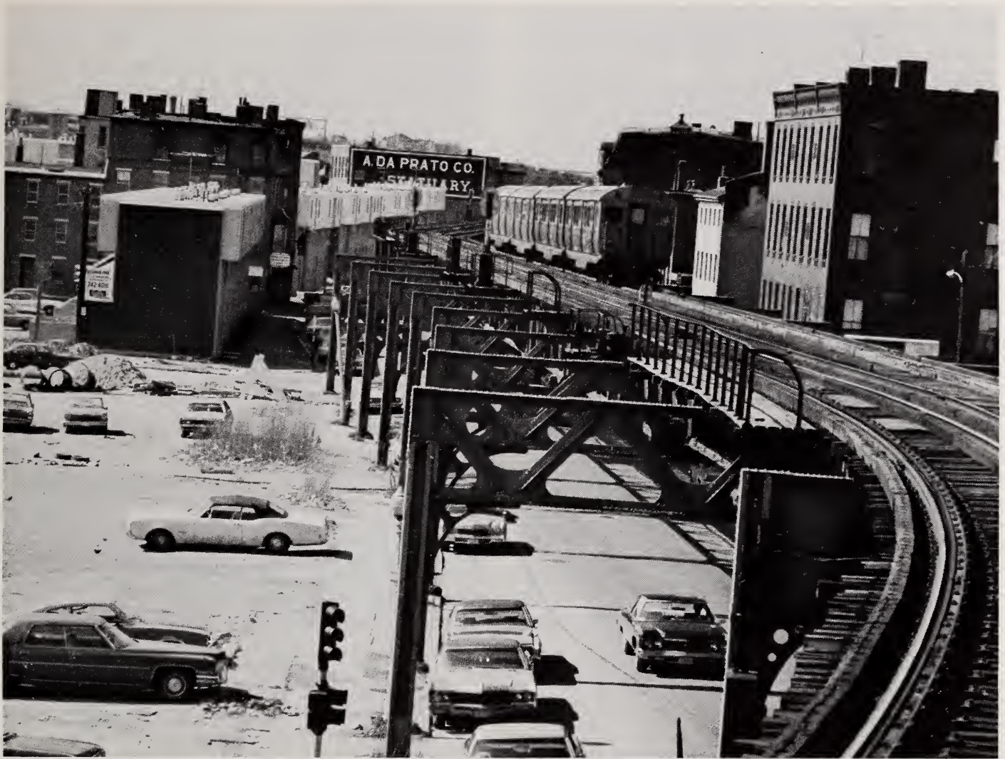
Noise levels for trains operated on elevated structures can be as much as 20 dBA higher than for trains operated at grade.
