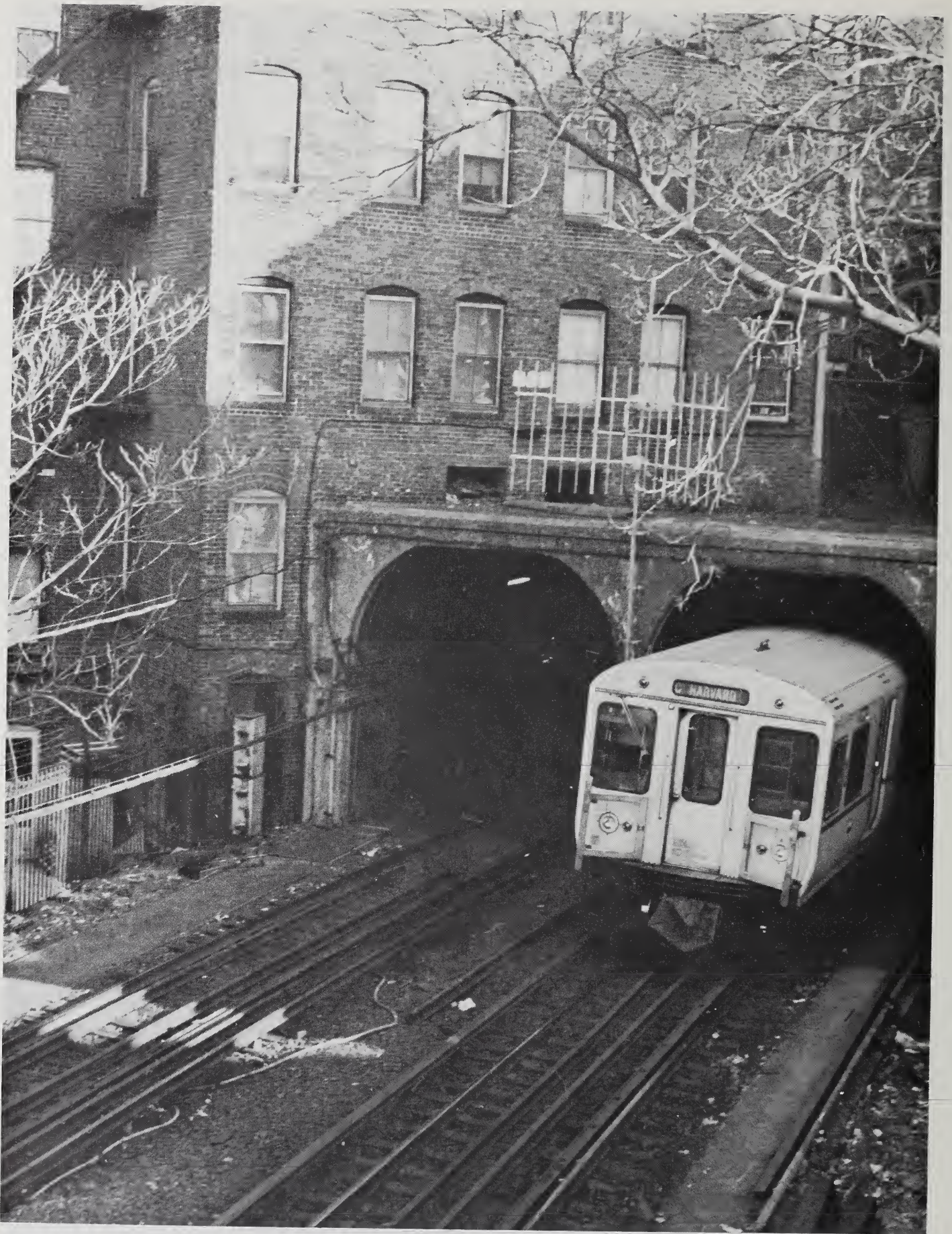
Train operations cause surrounding buildings to vibrate.
