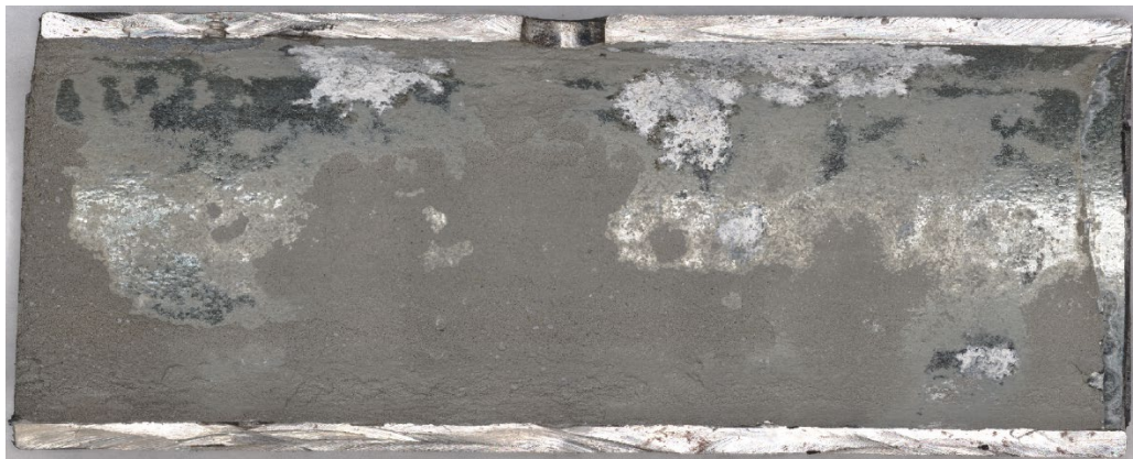
Figure 5-9: Inside view of the galvanized duct from Tendon 10 made with grout mixed from a 3.5% NaCl by weight of water solution ( w/c = 0.28 ).
