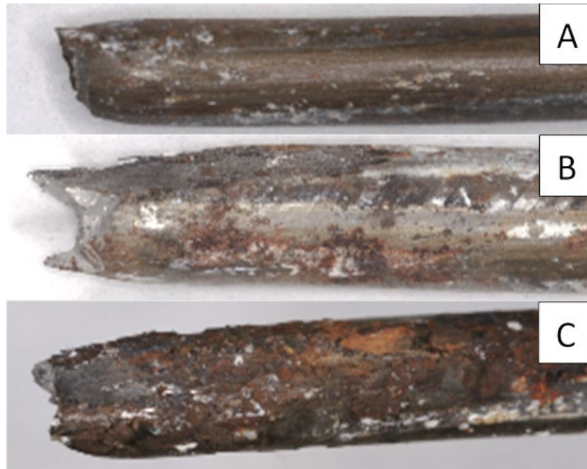
Figure 3-7. Example of (A) strands that have no corrosion, (B) mild corrosion, and (C) moderate corrosion.
