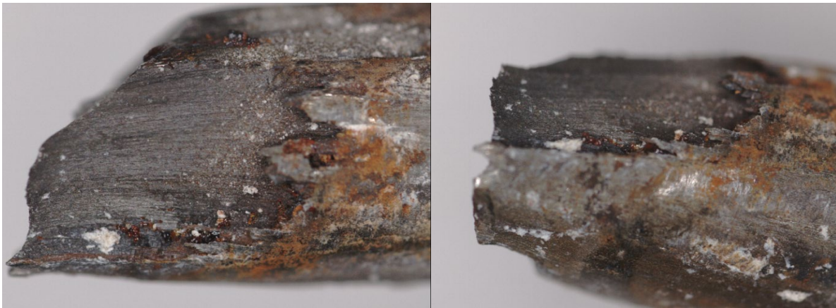
Figure 3-5. Example of a single wire with shear cracking at the fracture end.
