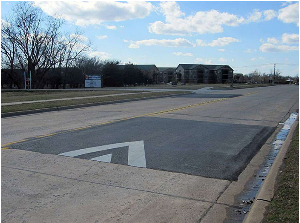
Figure 42 – Speed Table with Offset Design
