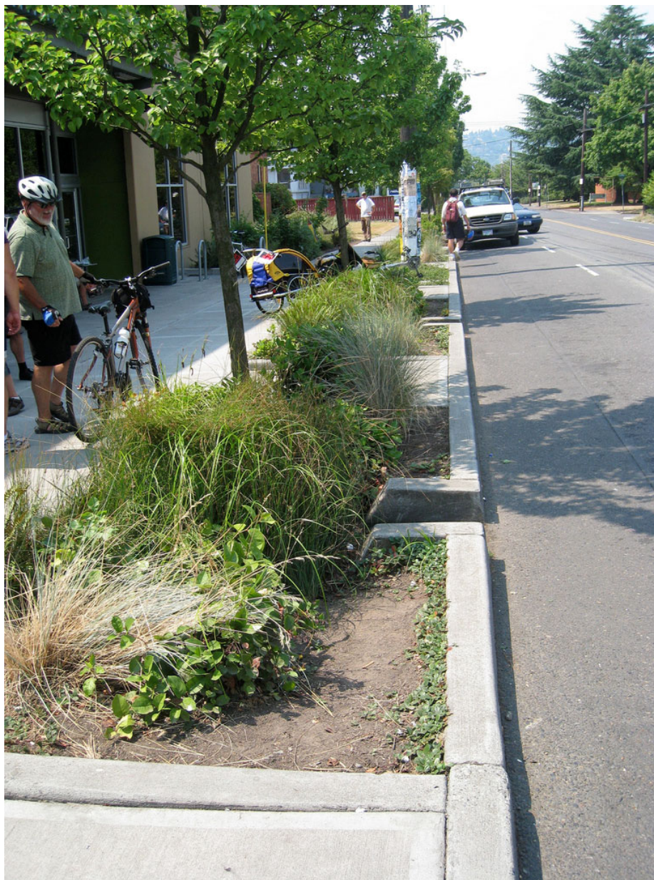
Figure 39 - Example of a Bioswale in Portland, OR
