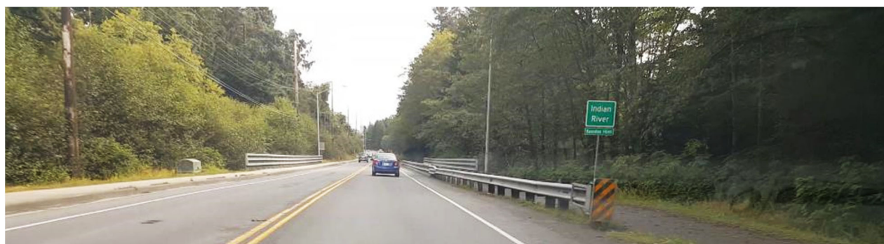
Figure 26 - EB multi-use path at Indian River bridge
