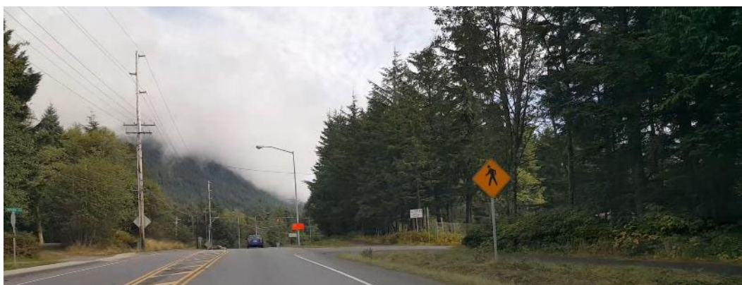
Figure 17 - EB SMC Road approaching Sisters Lane
