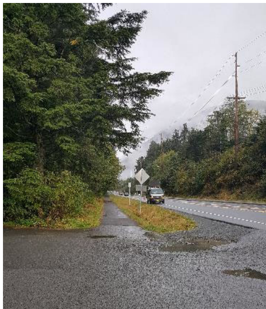
Figure 29 - Sawmill Creek Road at Sitka National Park Lot
