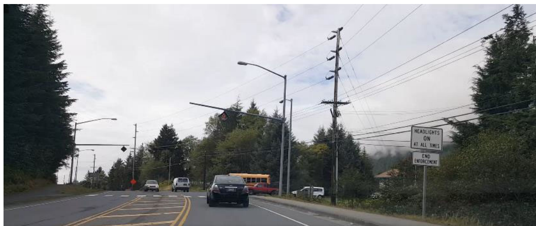
Figure 22 - WB Sawmill Creek Road at Indian River Road
