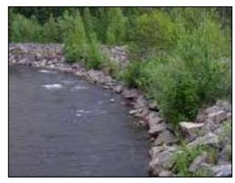
Riprap would be placed along streambanks to control the flow of Blacktail Creek, stabilize the banks, and prevent further erosion on Roosevelt Drive.
