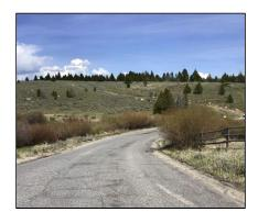
Between MP 2.2 and 2.4 there is an scurve with tight combination horizontal/vertical curves. The steep cut slope, vegetation, and parking along the road limits sight distance at this location.
