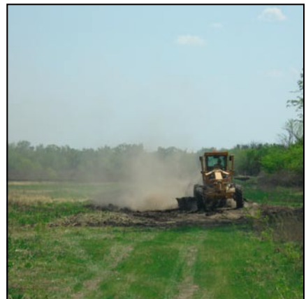
Road construction at Flint Hills NWR.
