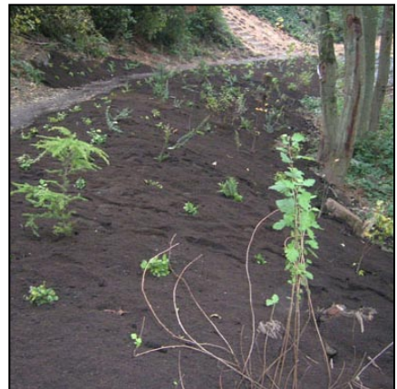
A decommissioned roadway is restored with native vegetation.
