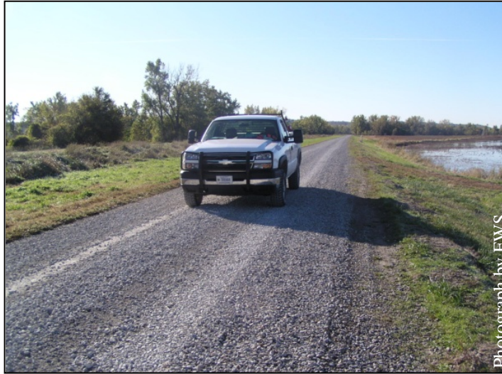
Figure 30. Squaw Creek NWR Project – The after
