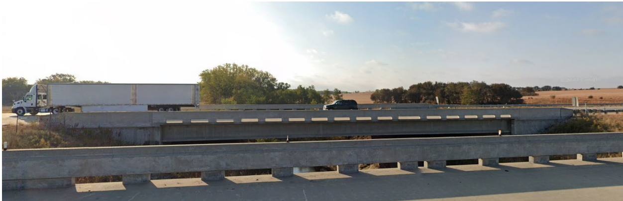
Figure 8.1 Prestressed Concrete Simple-Span Bridge (S080 41653) (Google Map, 2023)
