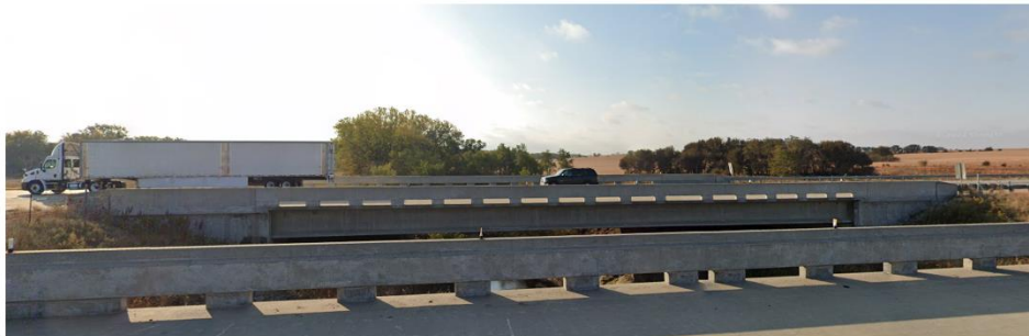
Prestressed concrete bridges (S080 41653 )
