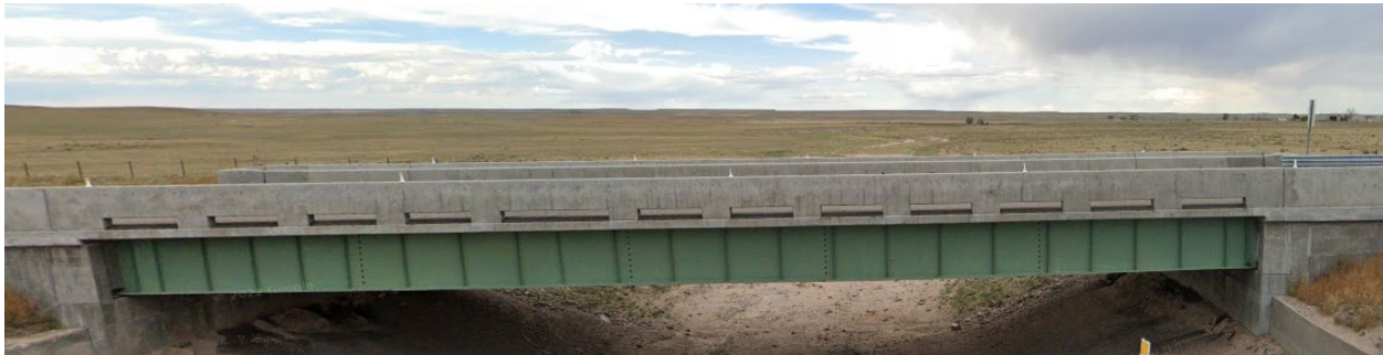
Figure 8.13 Steel Welded Plate Girder Simple-Span Bridge (S080 00526) (Google Map, 2023)
