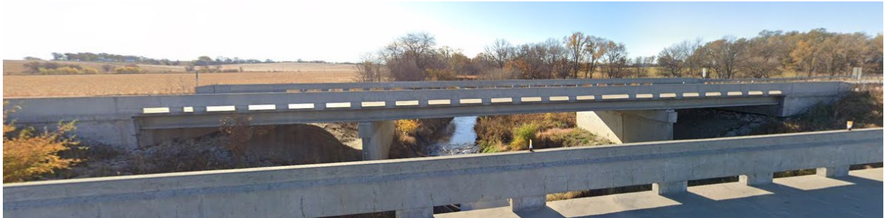
Figure 8.7 Prestressed Concrete Continuous Span Bridge (S080 41465) (Google Map, 2023)
