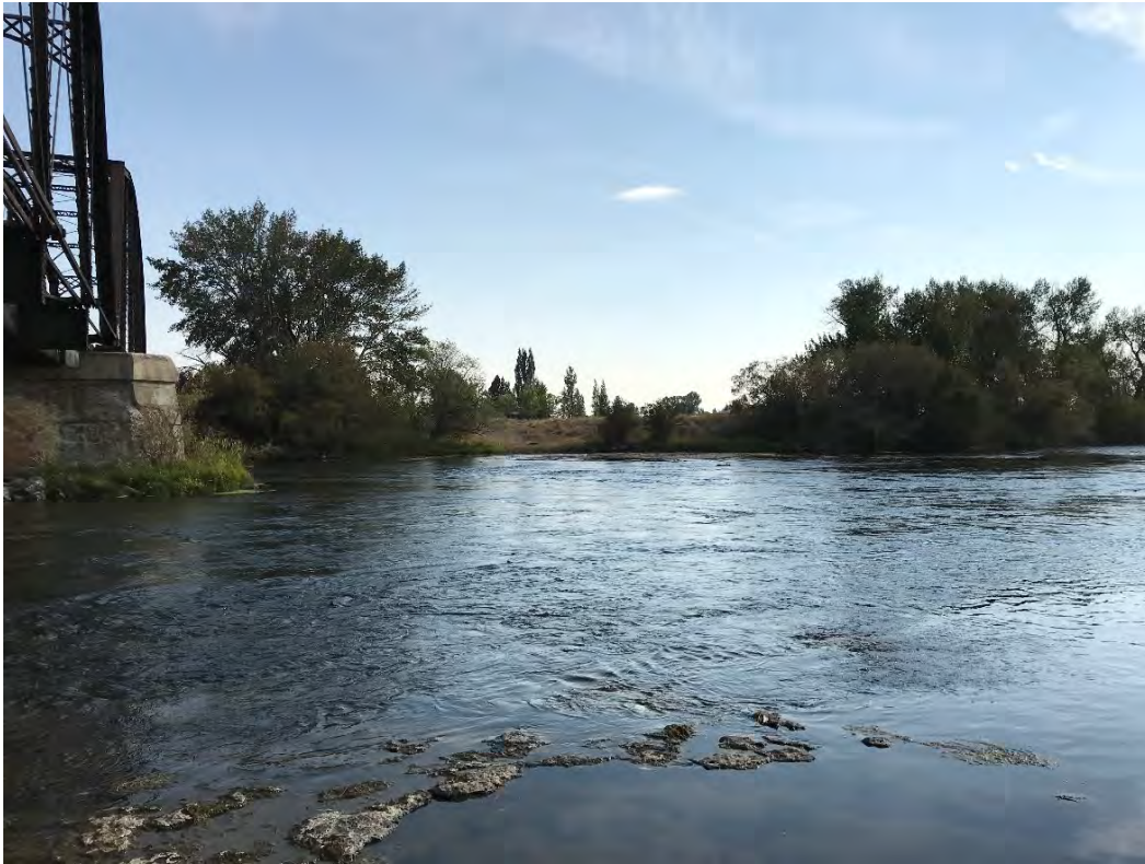
Picture 11. Facing south bank from downstream of existing rail bridge.
