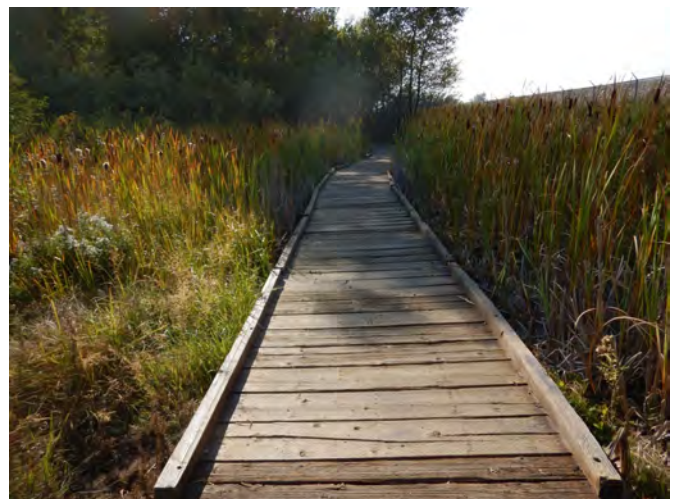
Boardwalk on North Side of River
