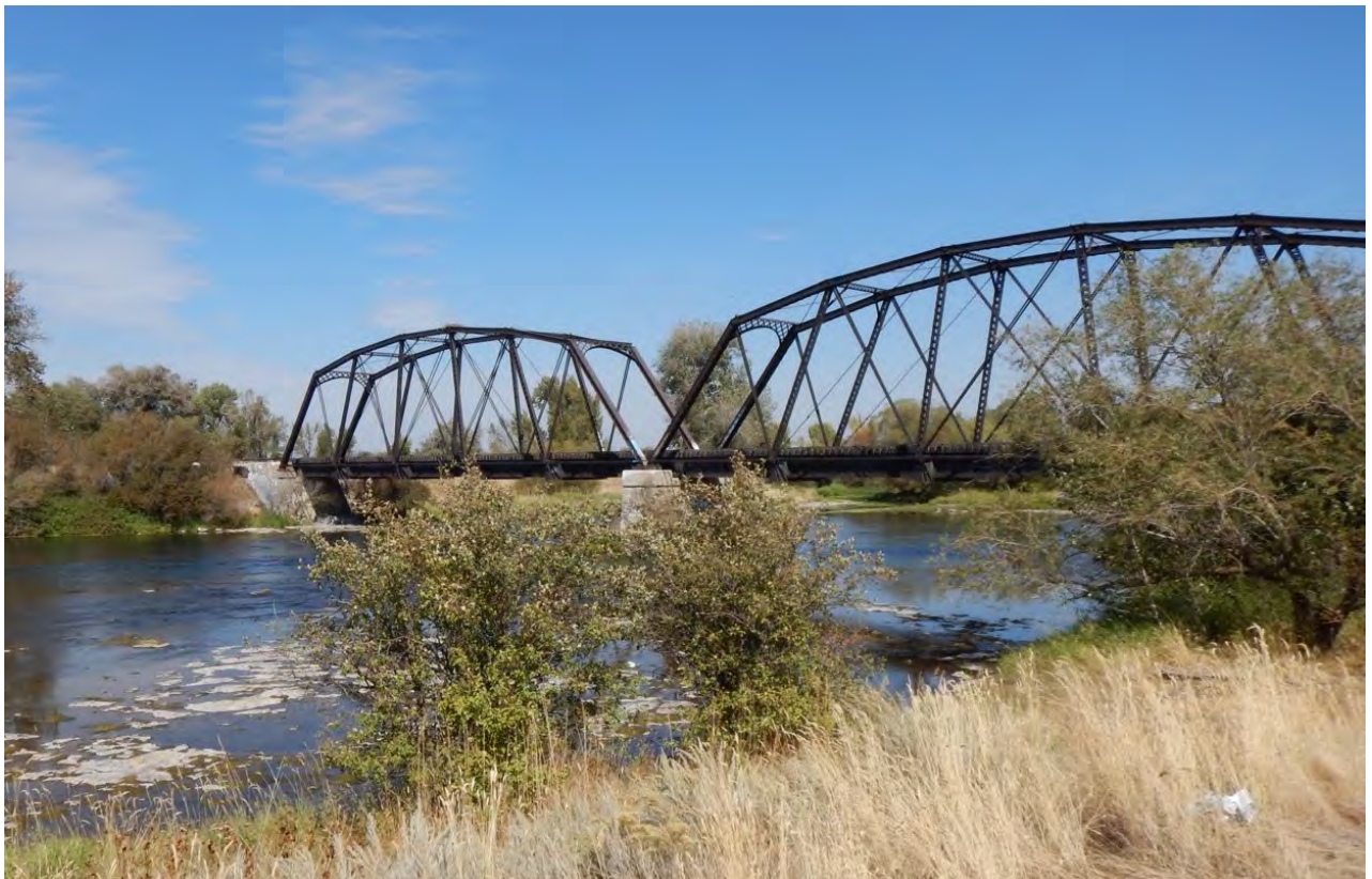
Existing Henry's Fork Pegram Truss Railroad Bridge
