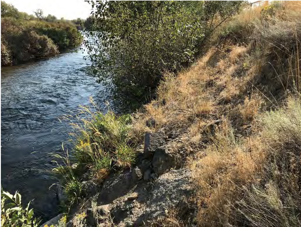
Picture 7. Bank stabilization performed ~10 years ago consisting of riprap placement and revegetation.
