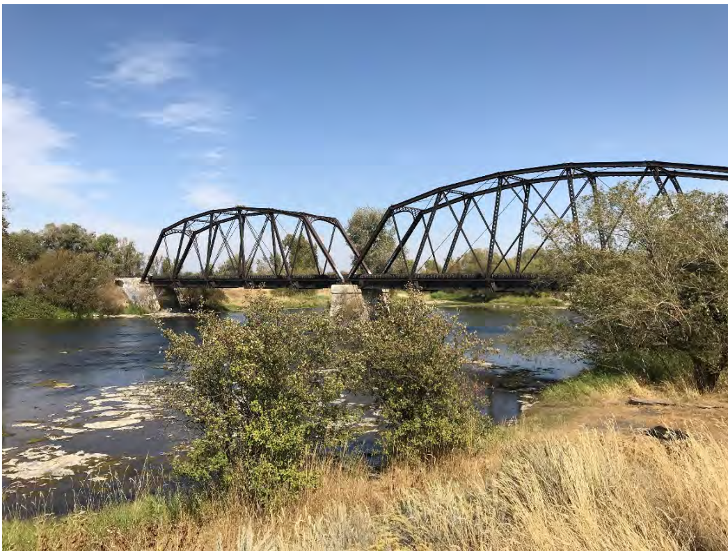
Picture 12. View of existing rail bridge from south bank.
