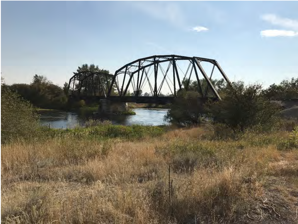
Picture 9. View of existing rail bridge from north bank.
