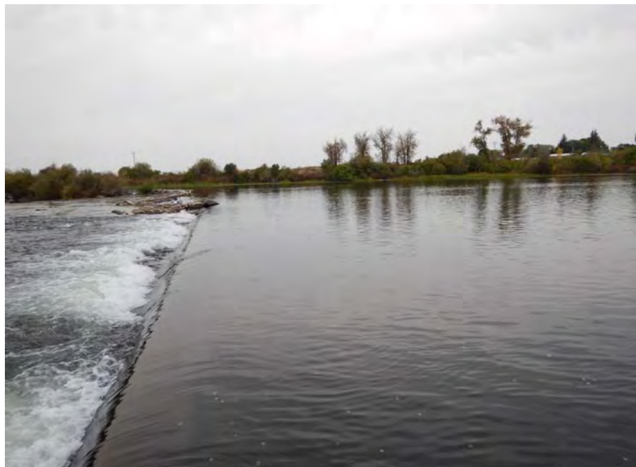
Diversion Weir at Northeast End of Study Area
