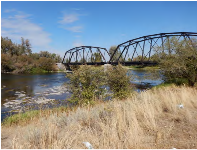
Henry's Fork Railroad Bridge
