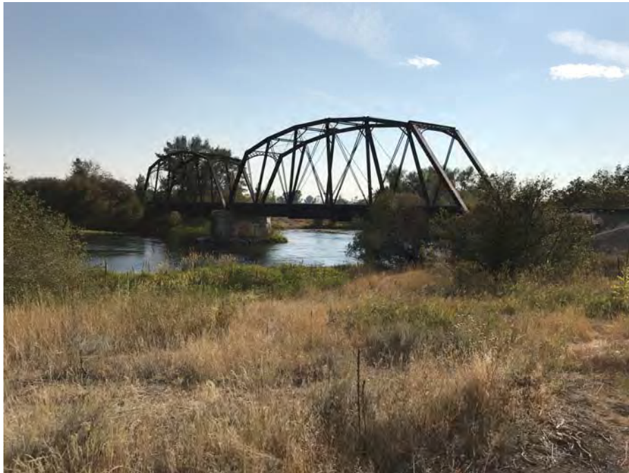
Historic Pegram Two-Span Truss Railroad Bridge
