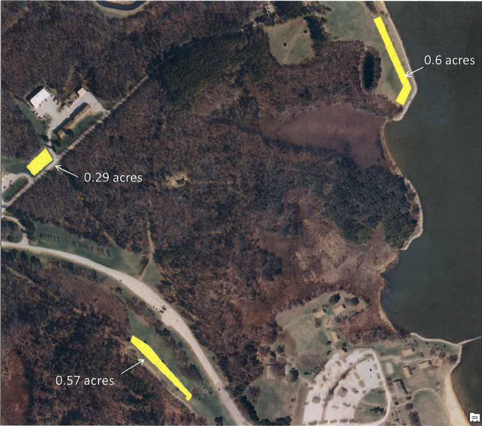
Tree Planting Areas to be Designed, Constructed, and Maintained by DNR for MDOT SHA CREDIT
