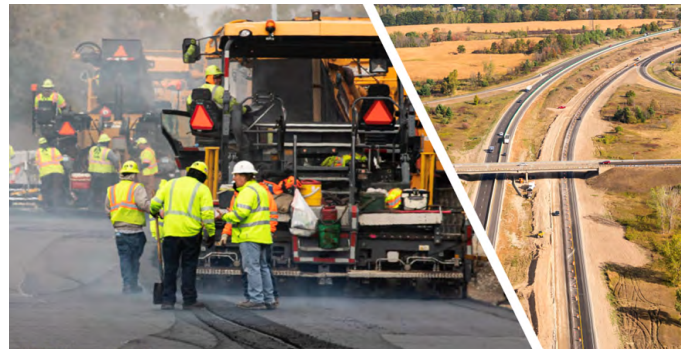
Using two pavers in close formation was found to be an important strategy for increasing the durability of asphalt roads.
