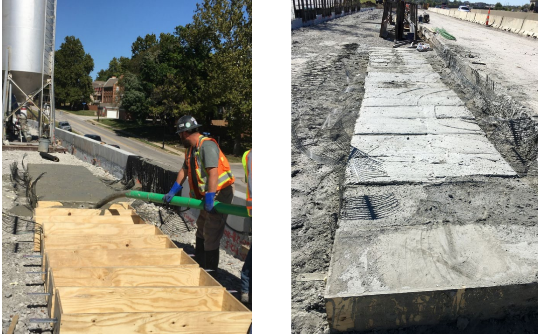
Figure 4.4: Pullout Specimens Cast on a Project Site
