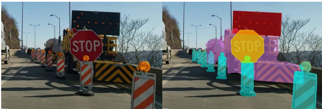
Figure 2: Left shows an example image of a work zone. Right shows an example with objects of interest that have been manually segmented by polygons. The polygons are overlaid with a unique color. Each segmented object is outlined with a solid line if it is not occluded and a dashed line if it is occluded.
