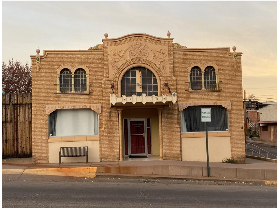
Figure 45. Separation between sidewalk and roadway; Silver City, New Mexico.
