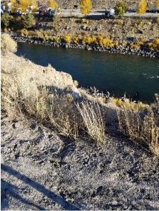
Figure 7 Mile 0.75. Erosion on the fill side above the Yellowstone River.
