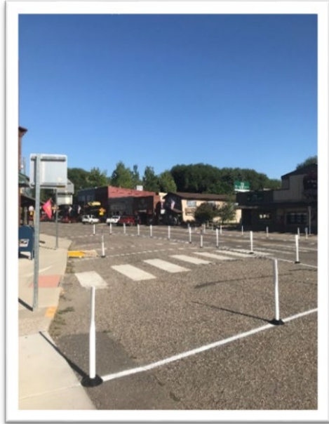
Figure 5. 1st Street Crosswalk
