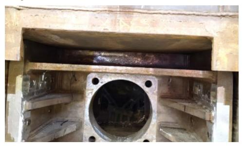
Figure 108. Contact between the Top of the Sliding Lug and the Top of the Draft Pocket
