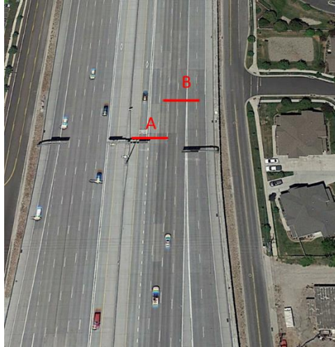
Figure 4.5 Example of Undersized Segment
