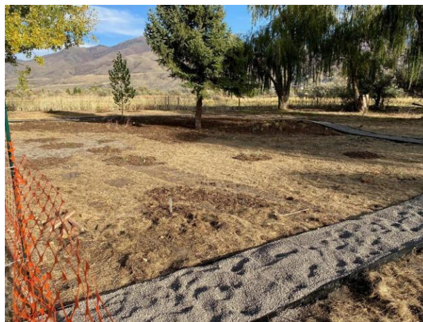
Figure 2.0-5 Walking path with chip seal material
