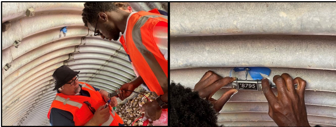
Figure 5.25. Strain gage installation.
