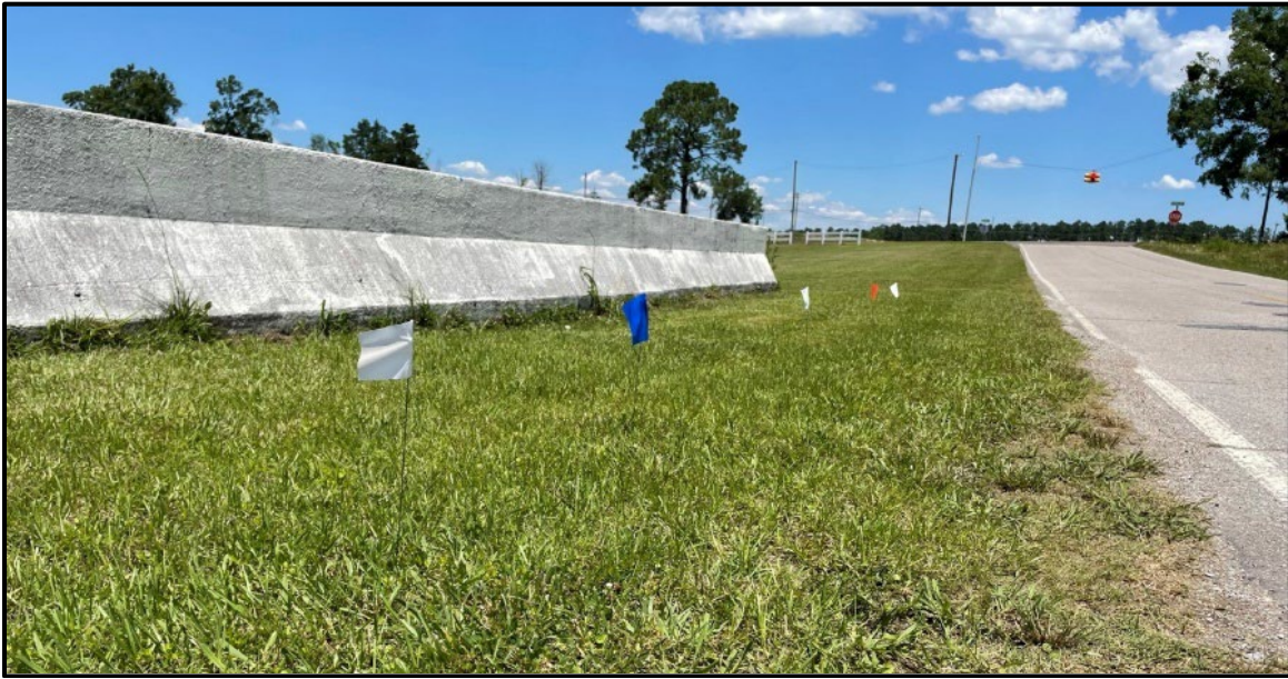
Figure 5.23. Signal flags located at the Bain's Gap Road culvert.
