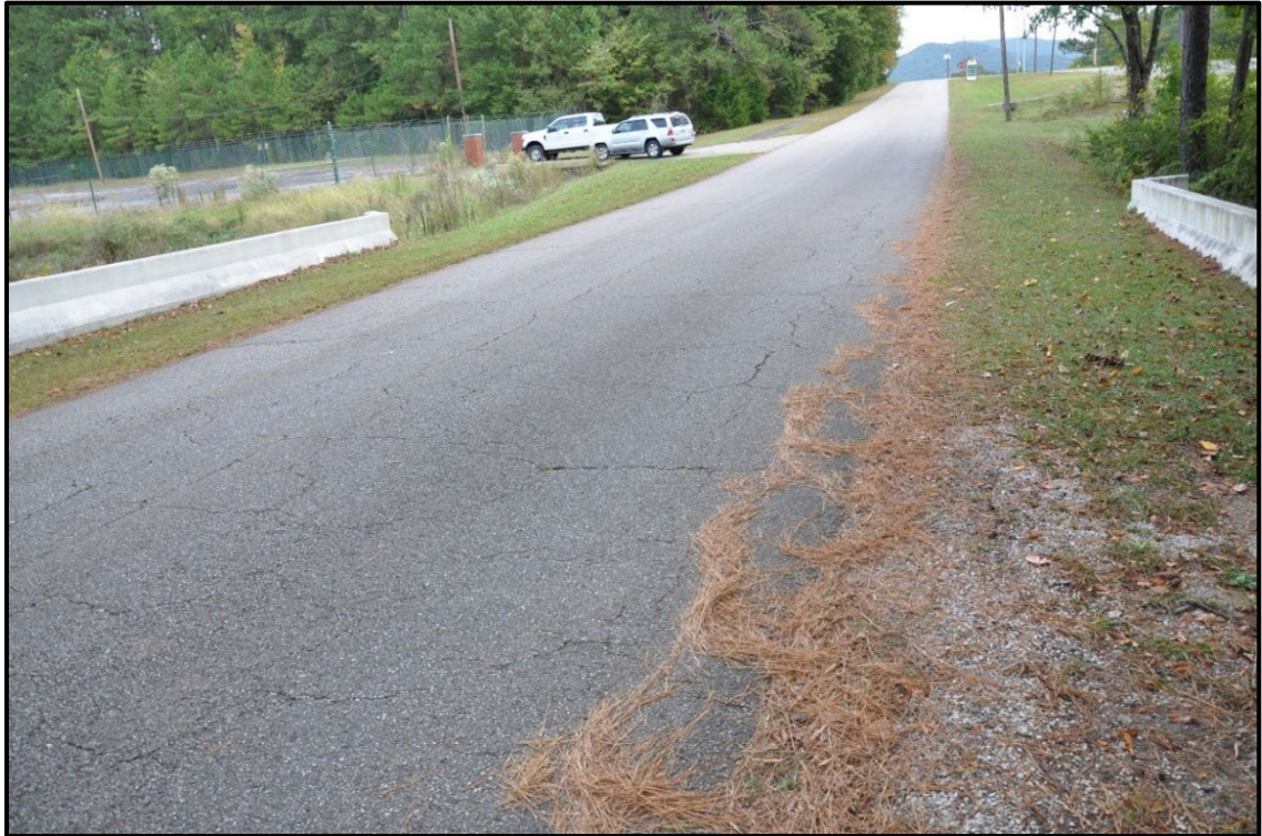
Figure 4.15. BIN 20441 road surface.
