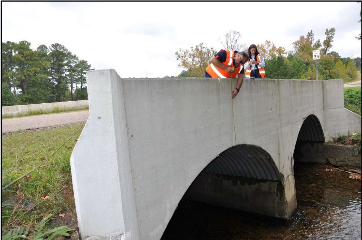
Figure 4.25. October 16, 2020 site visit.
