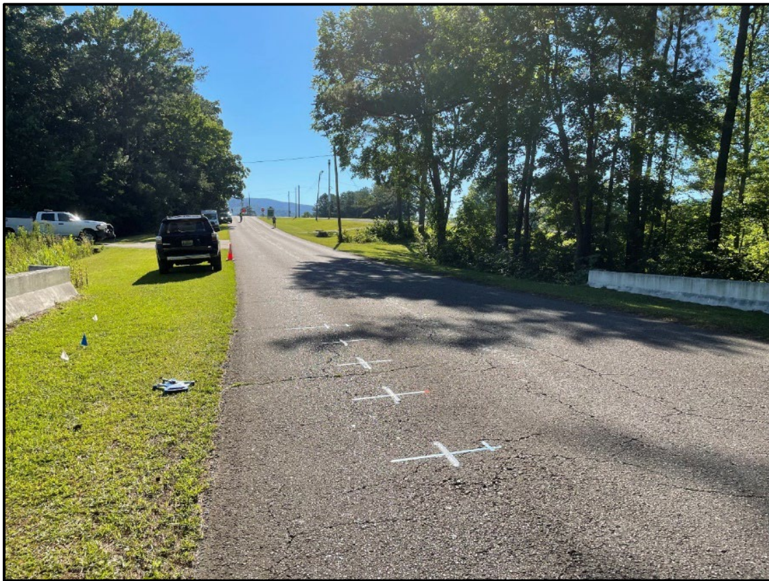
Figure 5.24. Truck stopping points located at the Berman Road culvert.
