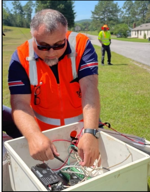
Figure 5.30. Connection of strain gages and potentiometers to the datalogger.
