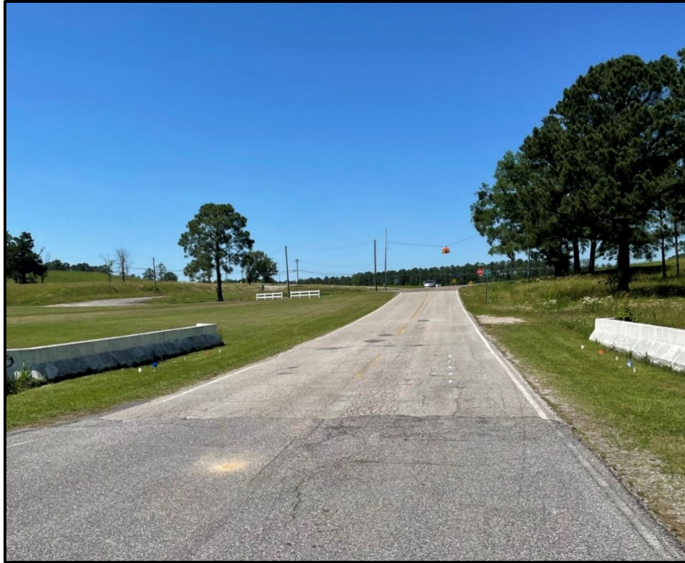
Figure 5.3. BIN 20433 longitudinal view.
