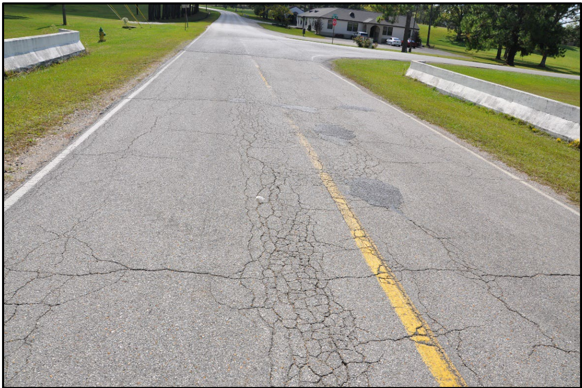
Figure 4.12. BIN 20433 road surface.
